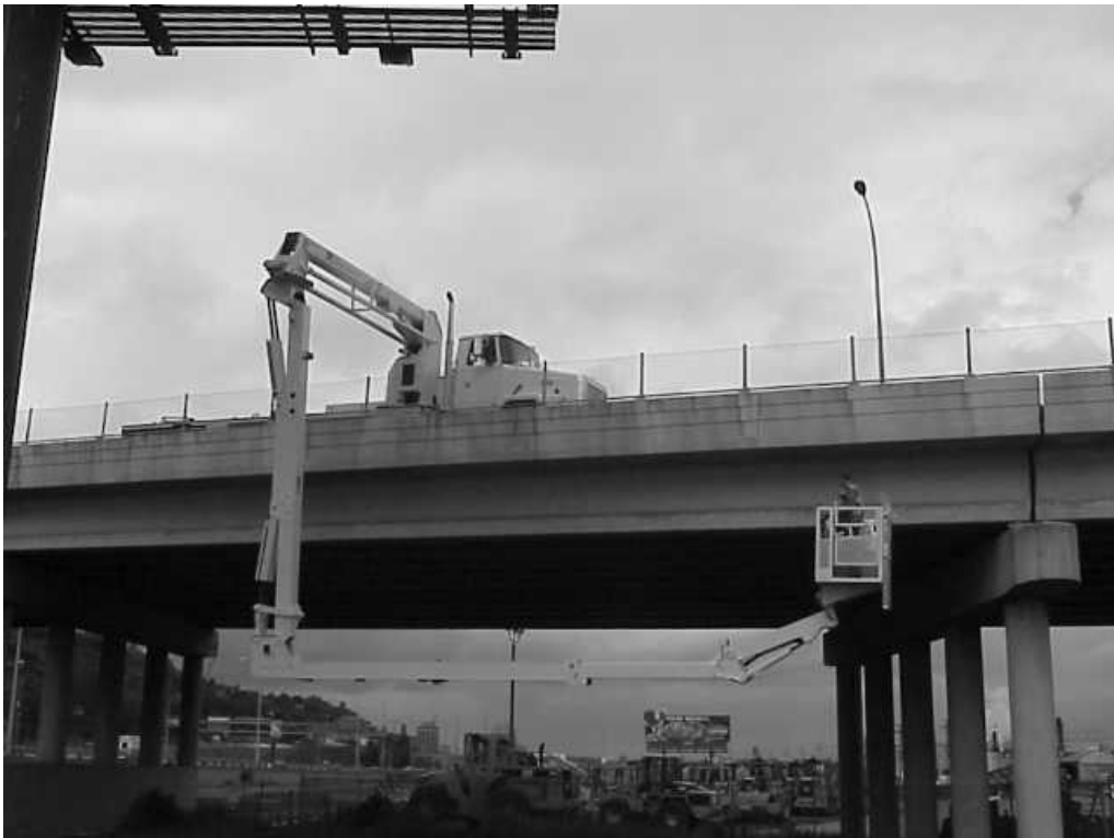
BOOMS MAY NOW BE MOVED INTO THE DESIRED POSITION
