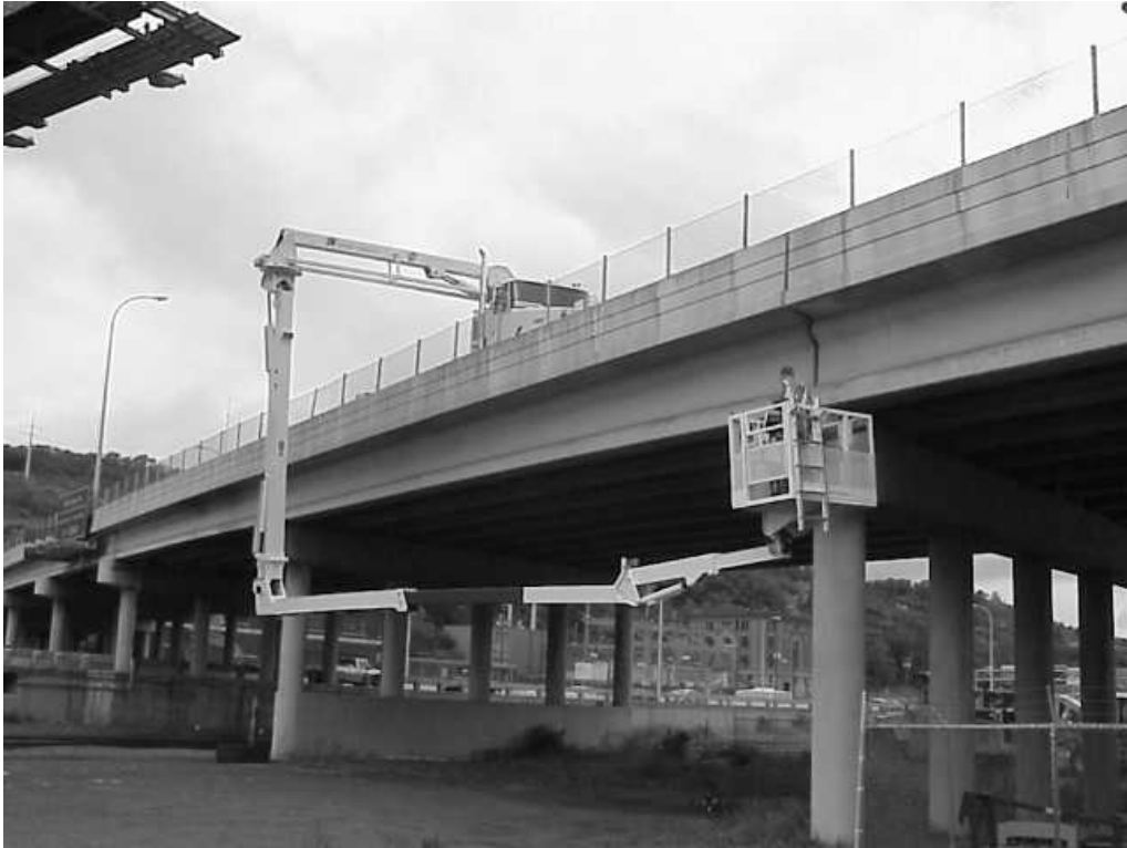
BOOMS #3 & #4 MAY BE TELSCOPED OUT ALONG SIDE OF THE BRIDGE
