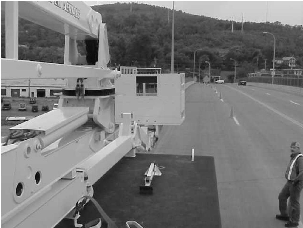
BOOM #4 IS LOWERED AND EXTENDED
