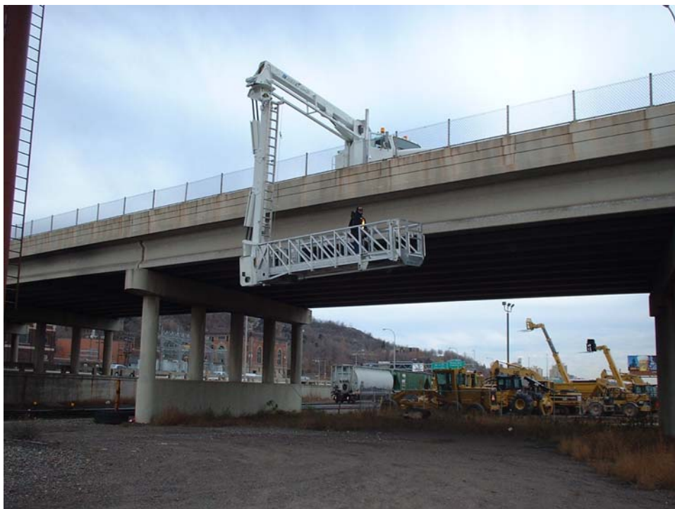
PLATFORM ALONG SIDE THE BRIDGE
