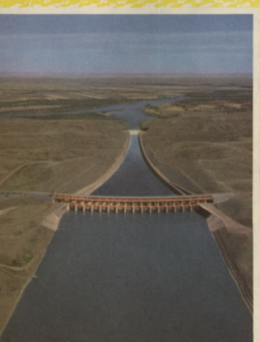
FORT PECK DAM Largest earth fill dam in the world. Fort Peck has tamed the mighty Mo by impounding the Missouri for a distance of 175 miles. Nearly four miles long, the dam measures 21,026 feet in length with a height of 250 feet, and has a concrete spillway a mile long. Fort Peck Lake has a shore line of 1600 miles and boasts a great variety of fish.
