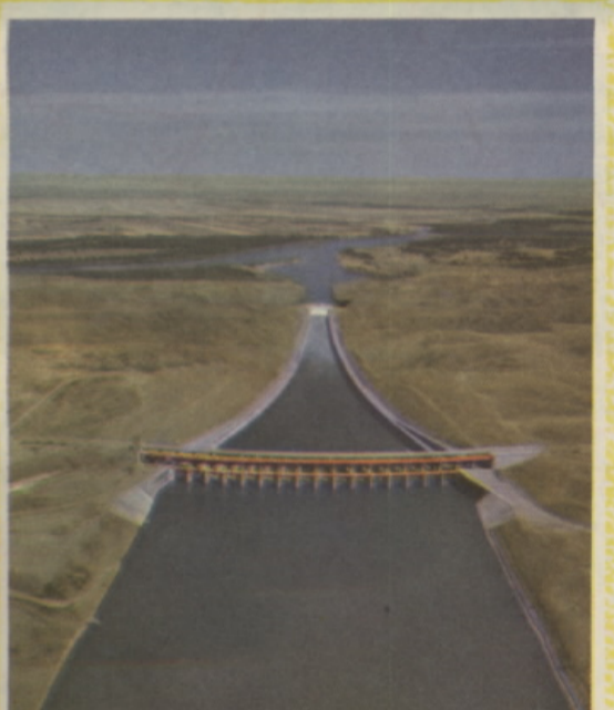
FORT PECK DAM SPILLWAY —An arresting feature of the mammoth Fort Peck dam in northeastern Montana is this spillway. The gate structure consists of 17 piers set in a curved line. Fort Peck has tamed the mighty Missouri by impounding the river into a lake 175 miles long. Many varieties of fish are caught in the lake.
