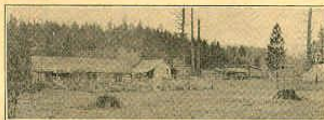
Historical Cabin On the Trail
