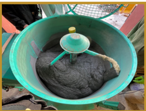
Figure 2: UHPC being mixed.
