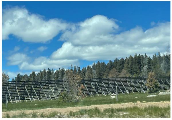
Drift Control - Snow Fences, Grading, and Snow
