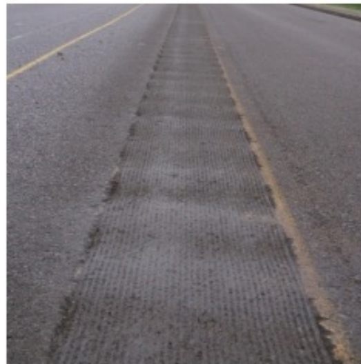
Source: Terhaar, et al. Sinusoidal Rumble Strip Design Optimization Study . Minnesota Department of Transportation, 2016.
