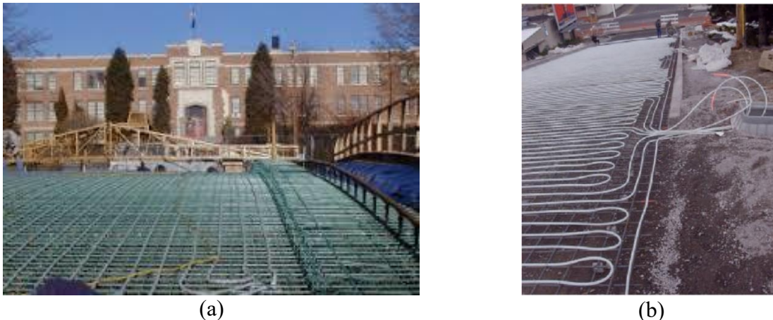
Figure 31. (a) Longitudinal closed loop on the bridge deck and (b) approach road loops in Klamath Falls, Oregon (Boyd, 2003)
