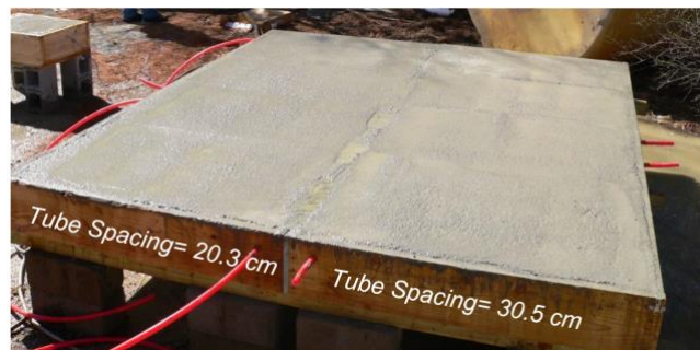
Figure 8. Photograph showing the poured concrete into the deck frame works (Bowers, 2016)
