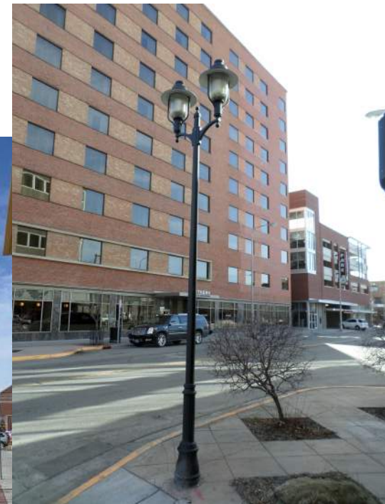
DOWNTOWN BILLINGS PEDESTRIAN LIGHTING
