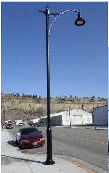
DECORATIVE LIGHTING WITHIN EAST BILLINGS URBAN RENEWAL DISTRICT
