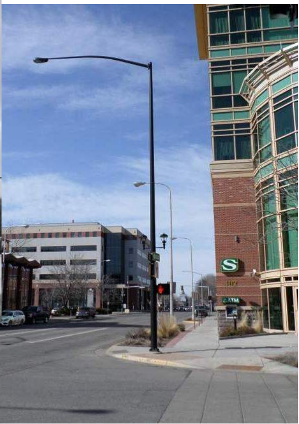
MDT STANDARD LIGHTING WITH BLACK POWDER COATING (4th Ave. N./ BROADWAY)
