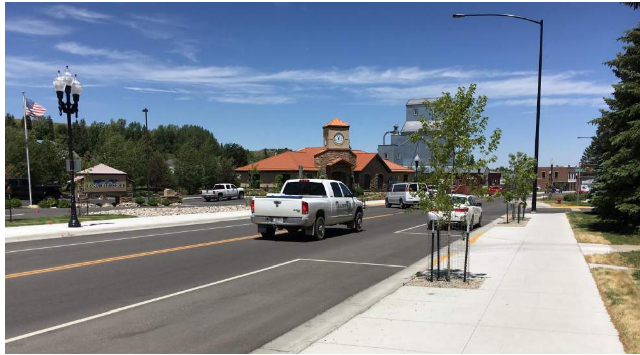
MDT STANDARD LIGHTING IN COMBINATION WITH DECORATIVE LIGHTING (RED LODGE)
