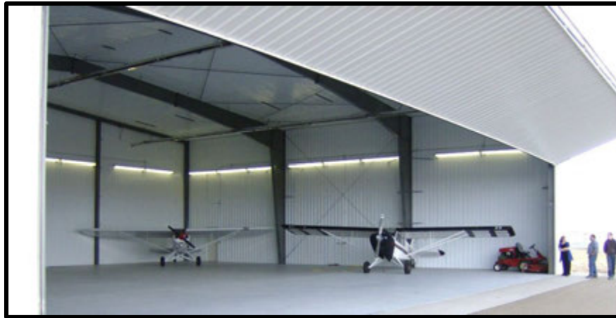
Figure 9.6: Hangar at Baker Municipal Airport
