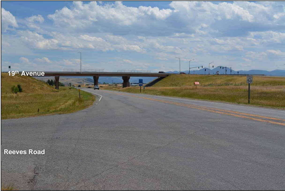
Photo 27: Looking east at Reeves Road (RP 3.1)
