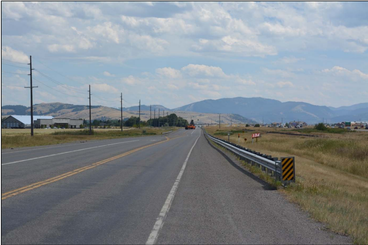
Photo 23: Looking east near Valley Center Spur Road (RP 25.6)
