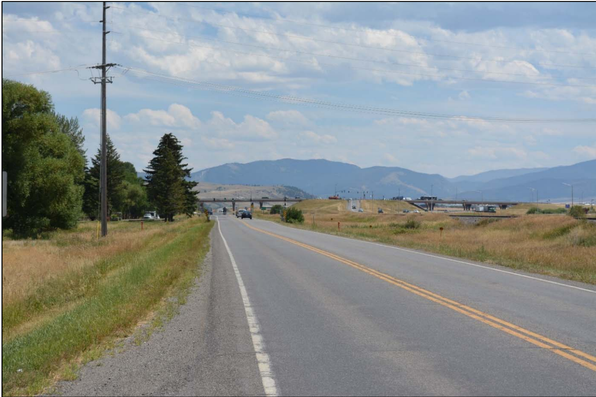
Photo 25: Looking east at RP 26.5
