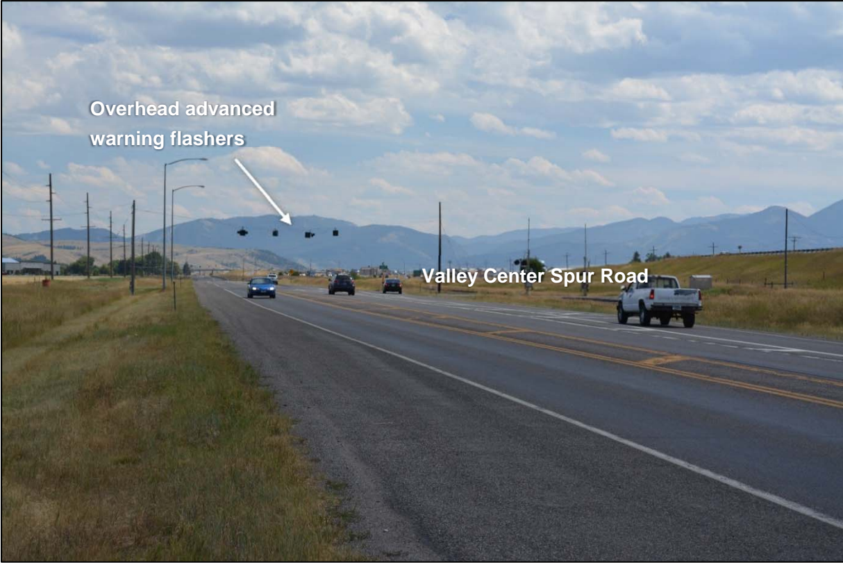
Photo 22: Looking east near Valley Center Spur Road (RP 25.4)
