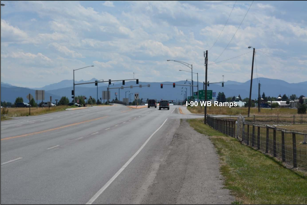
Photo 32: Looking south near Griffin Drive (RP 1.4)
