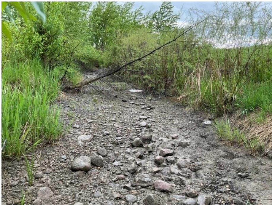
Photo 22a: View to the northwest of irrigation ditch ID-2a, Post A Canal.
