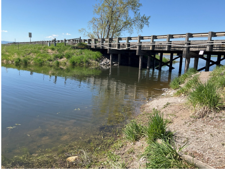
Photo 0: View to the southwest of the ID-1 Ninepipe Feeder Canal, flowing west under US 93.
