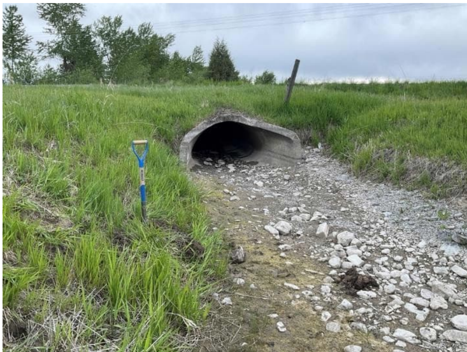
Photo 23: View to the south of potential wetland fringe along Post A Canal; no hydric soil indicators present (S-9).
