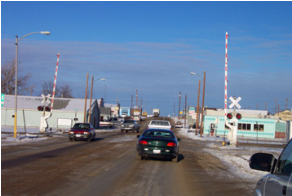
Existing at-grade crossing at Central Avenue (existing S-213) and BNSF tracks, looking northeast.
