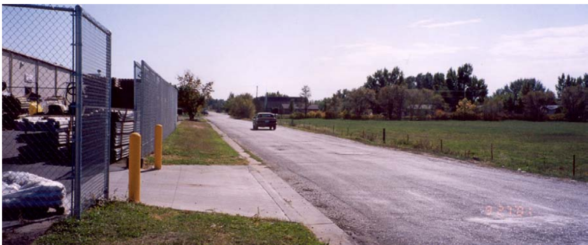
Stower St. at Moorehead Ave. (looking south down Moorehead)
