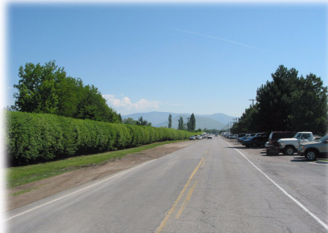
Photo B: Existing Old US 93 between Brooks and Reserve Streets would be widened to three travel lanes and a left-turn lane with addition of sidewalk and bike lanes (looking north on Old US 93 toward east).
