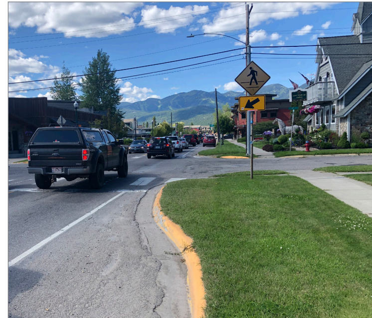
Curb bulbouts, like this one at Spokane Avenue/4th Street, reduce the crossing distance for pedestrians.
