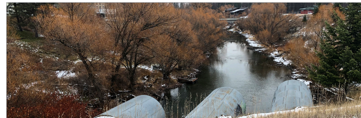
There are currently two Whitefish River crossings within the study area at Baker Avenue and Spokane Avenue. It is important to minimize impacts to fisheries, habitat, and wetlands at these crossings.
