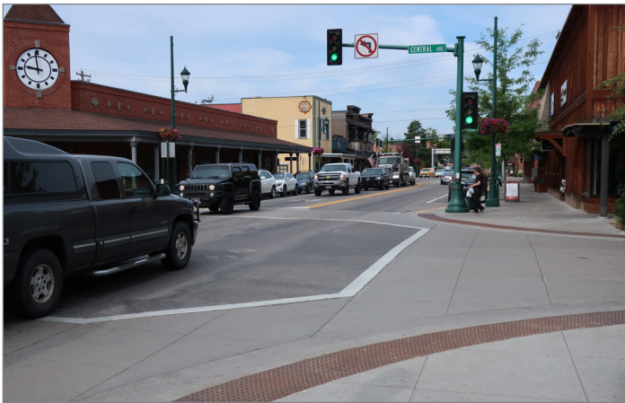
To improve safety at the 2nd Street/Central Avenue intersection, the signal timing could be modified to include leading pedestrian intervals or dedicated crossing phases.
