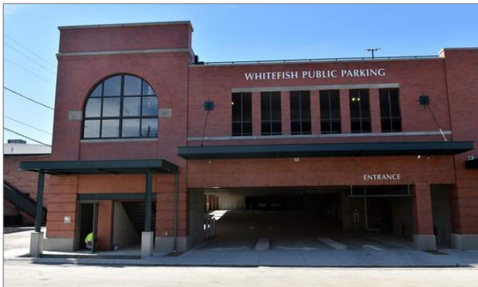
The City of Whitefish recently constructed a three story parking garage to provide additional parking for Downtown businesses and visitors.
