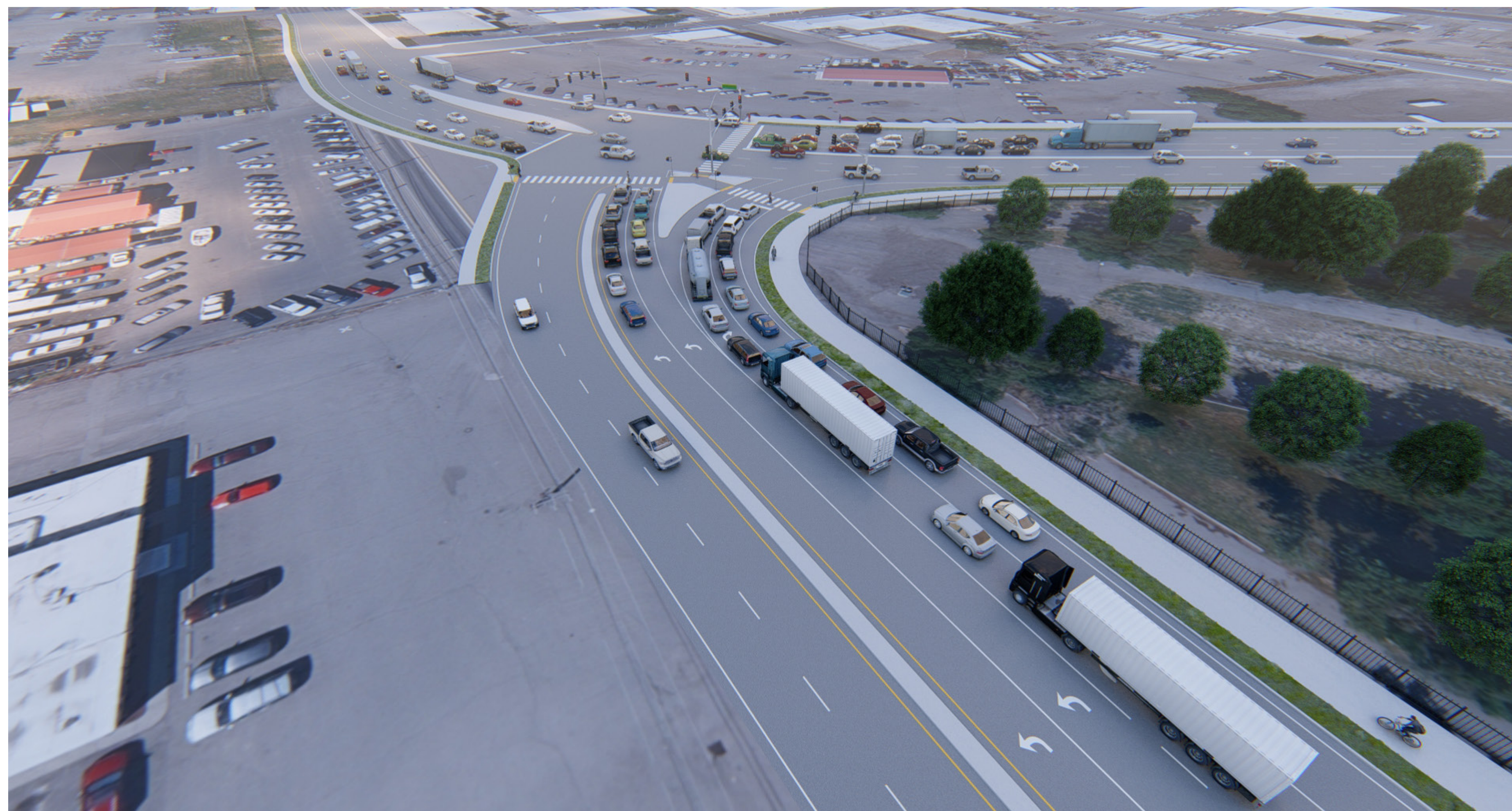
LOOKING WEST FROM 1ST AVENUE N
