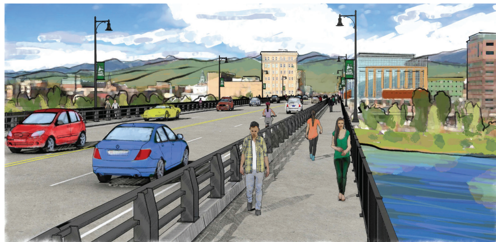
Figure 4. Bike Lane Option Looking North. This view represents a possible configuration where a bike lane would be provided adjacent to the traffic lane. A dedicated walkway would be provided for pedestrians with positive separation from the roadway. Either steel traffic railing (pictured here) or concrete barrier (Figure 5) would be provided between the walkway and roadway.
