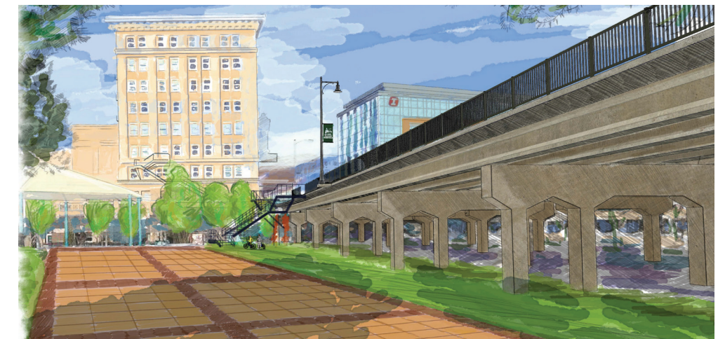
Figure 6. Caras Park Rendering. This view depicts how the intermediate bridge supports will be widened to the west over dry land. The existing stairs on the west side of the bridge will either be relocated to accommodate the wider bridge deck, or replaced at a similar location. Some modifications to the landscaping at Caras Park will be necessary to accommodate the bridge widening.
