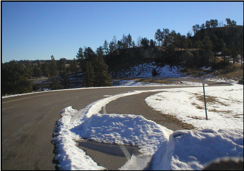
Photo 8. Acceleration ramp at Custer EB site.
