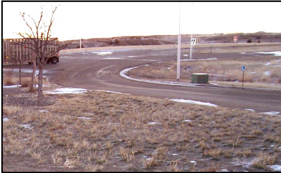
Photo 18. Acceleration ramp at Hathaway WB site.
