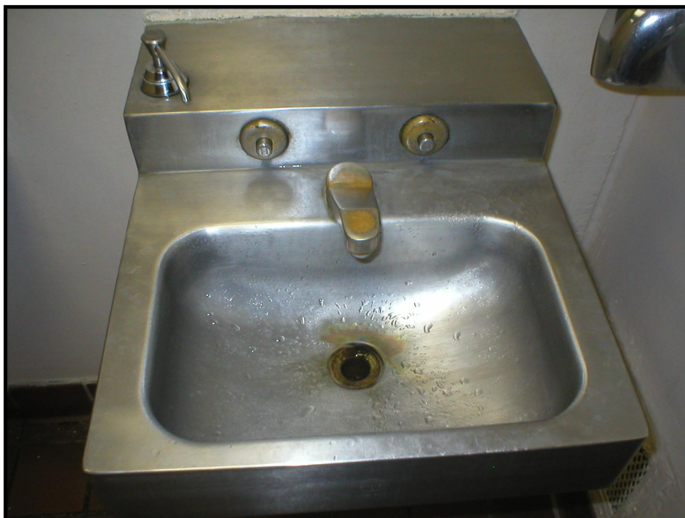
Photo 10. Rusted sink at Hysham EB site.
