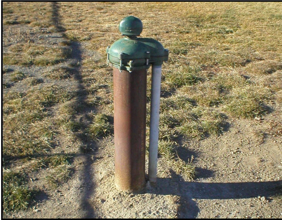
Photo 6. New Greycliff EB well head.
