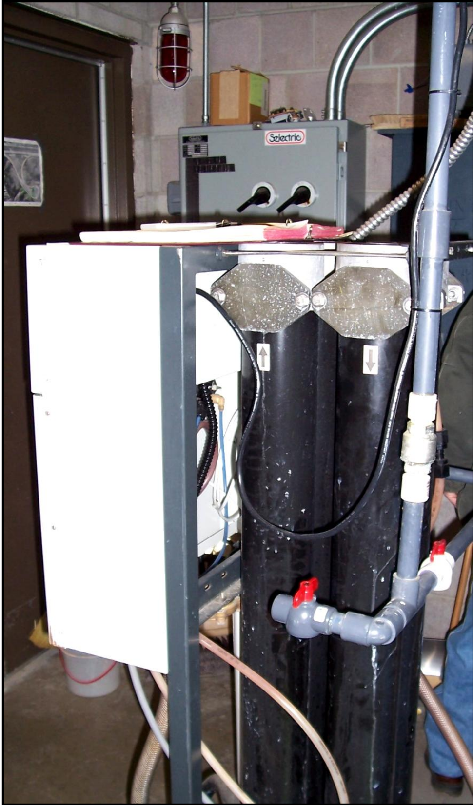
Photo 42. RO unit at Hathaway WB.
