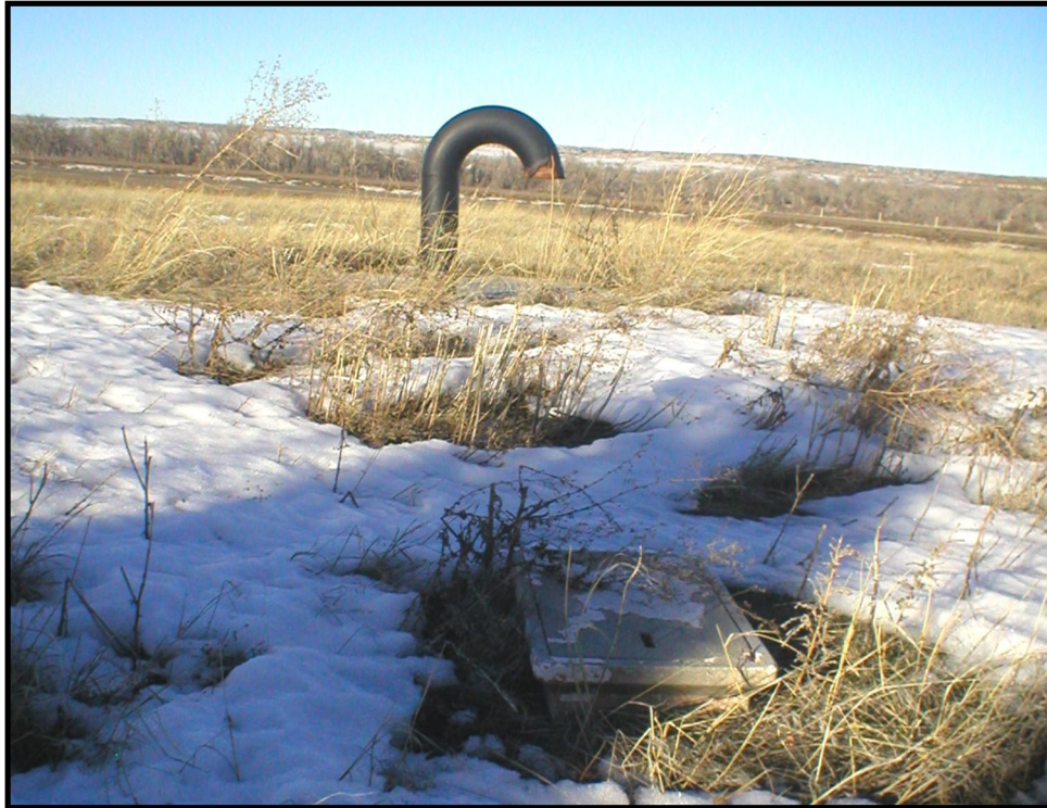
Photo 36. Septic tank at Hathaway EB.
