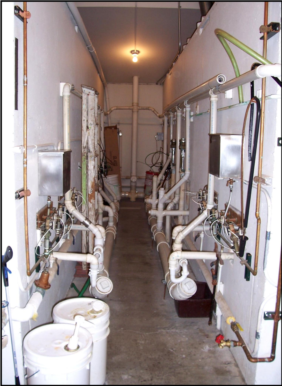
Photo 29. Water and Sewer Plumbing for Hysham WB.
