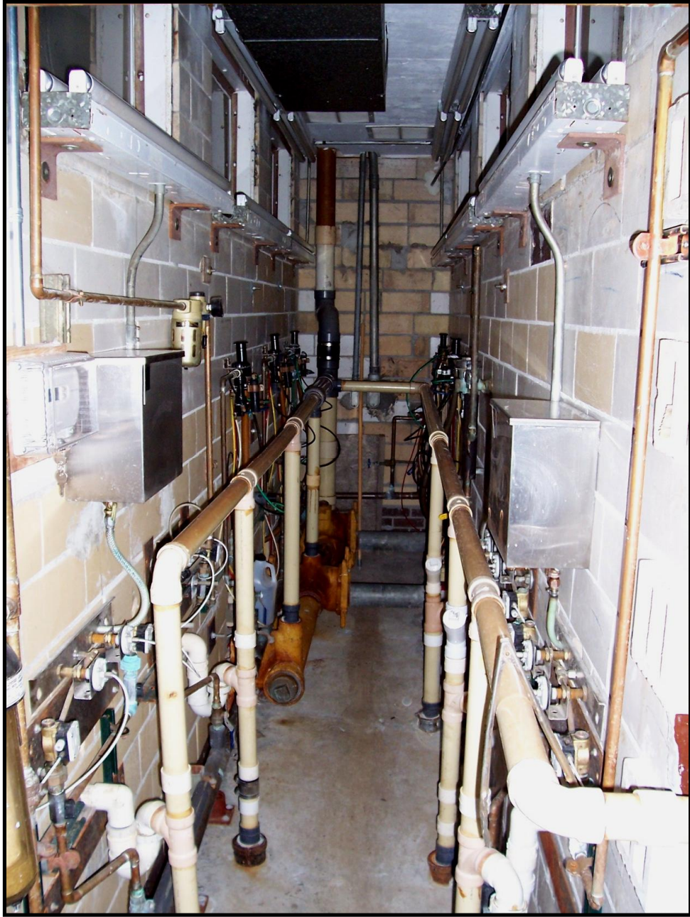
Photo 21. Water and Sewer Plumbing for Custer WB.
