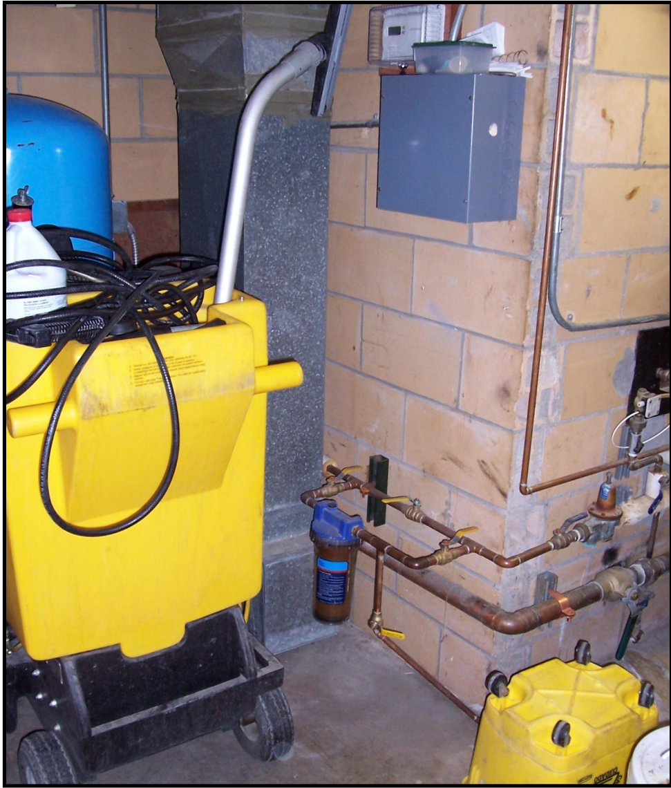
Photo 9. Cartridge Filter
