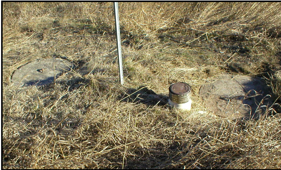
Photo 3. Septic Tank for Greycliff EB.
