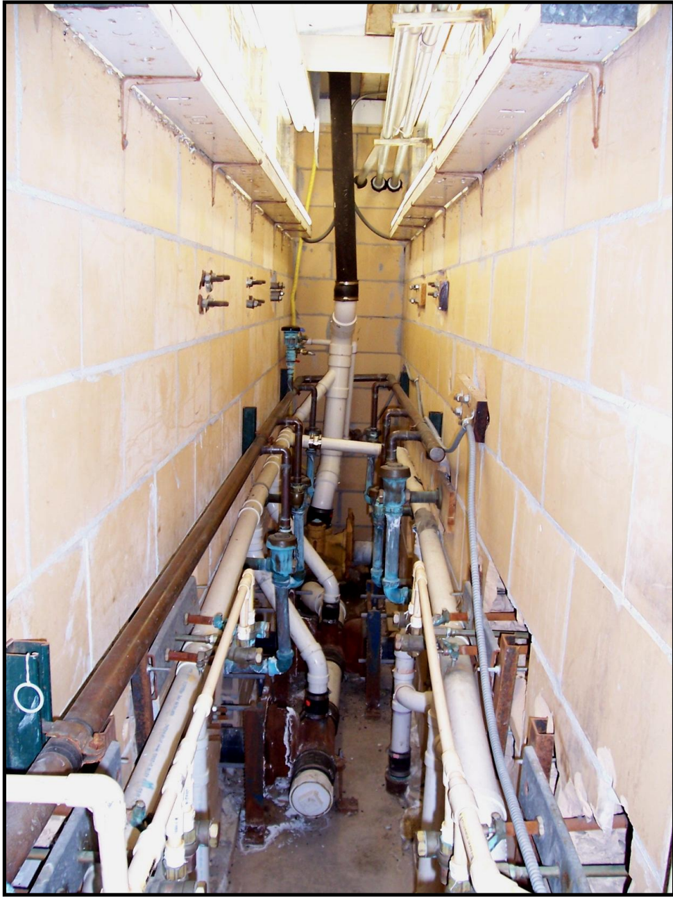
Photo 41. Water and sewer plumbing at Hathaway WB.
