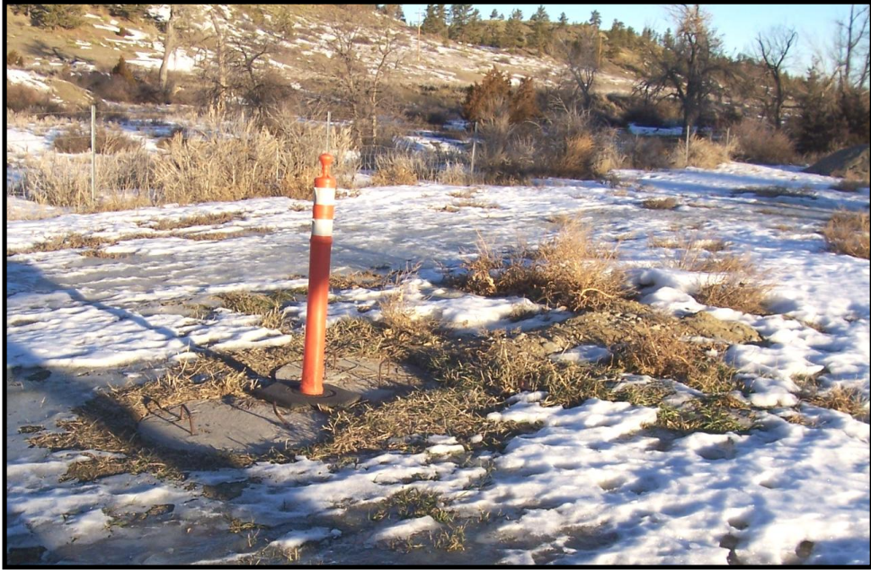
Photo 32. Septic tank for Hysham WB.
