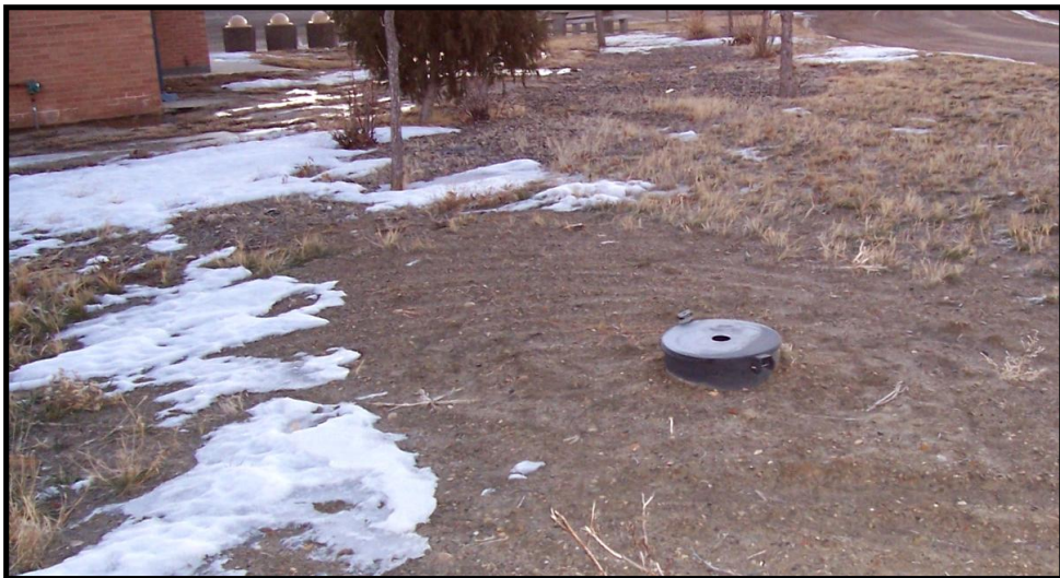
Photo 46. Underground propane tank for Hathaway WB.
