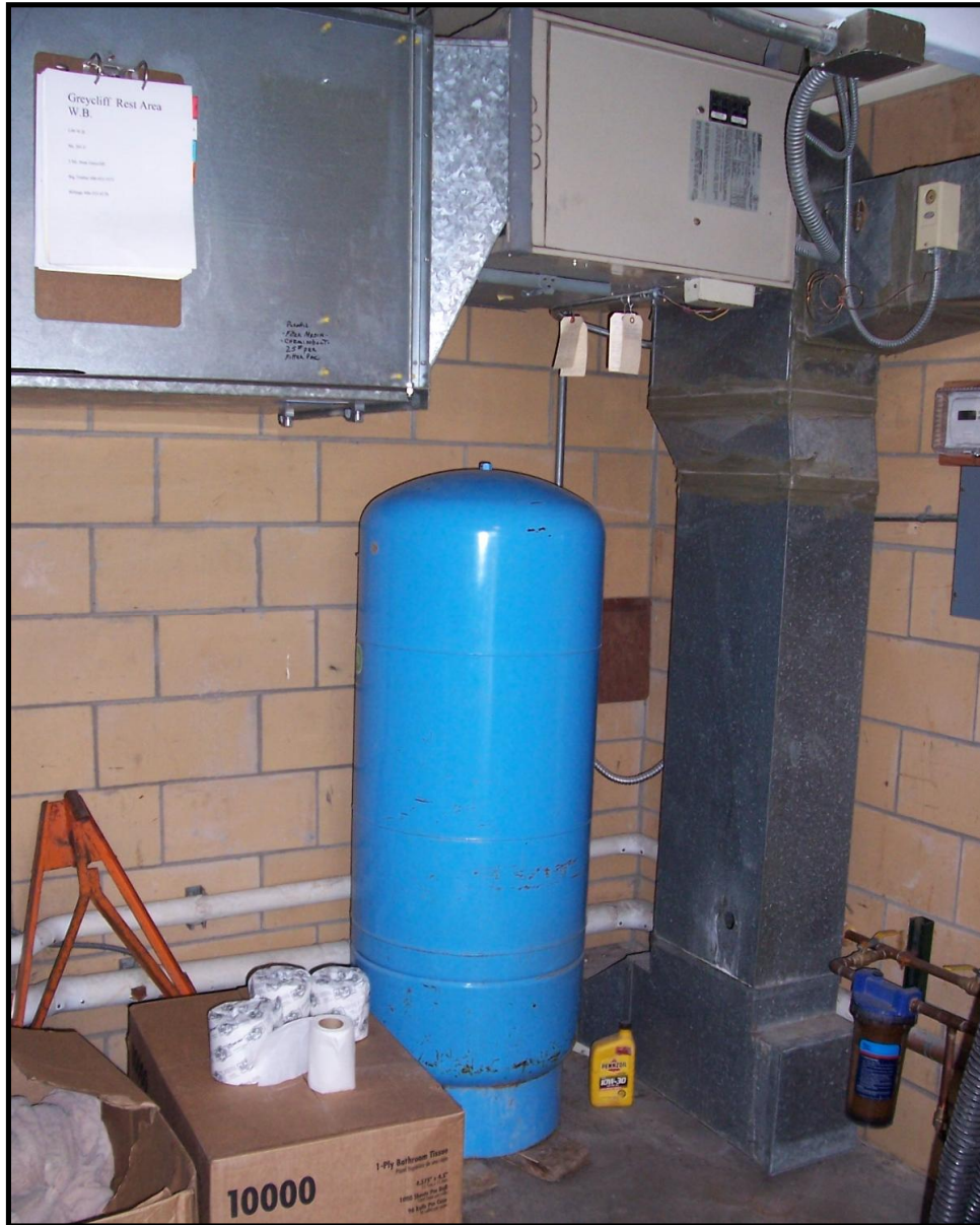
Photo 8. Pressure Tank
