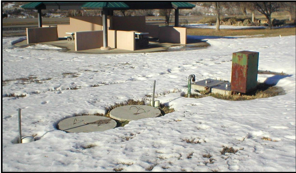
Photo 28. Septic tank and dosing chamber for Hysham EB.
