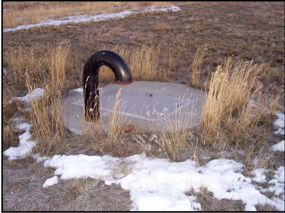
Photo 43. Sewer vent and sewer manhole for Hathaway WB.
