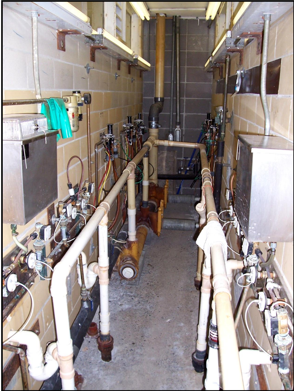
Photo 17. Water and Sewer Plumbing for Custer EB
