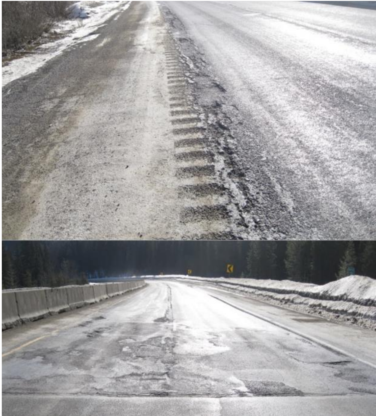
Figure 2 – Pavement distress visible at the surface, March 2020
