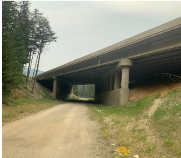
Local Access Bridge @ RP 5.2
