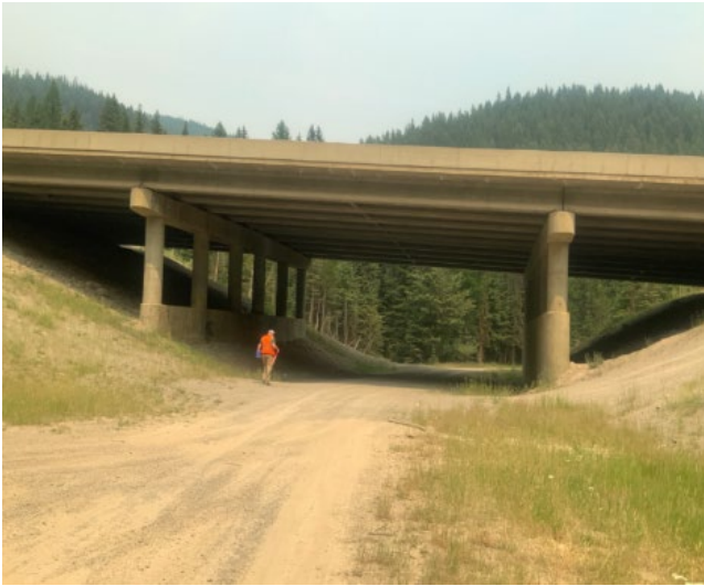
Local Access Bridge @ RP 1.9
