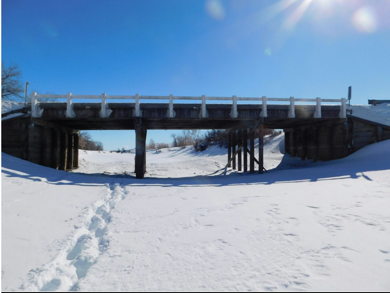
Bridge over Dodson South Canal
