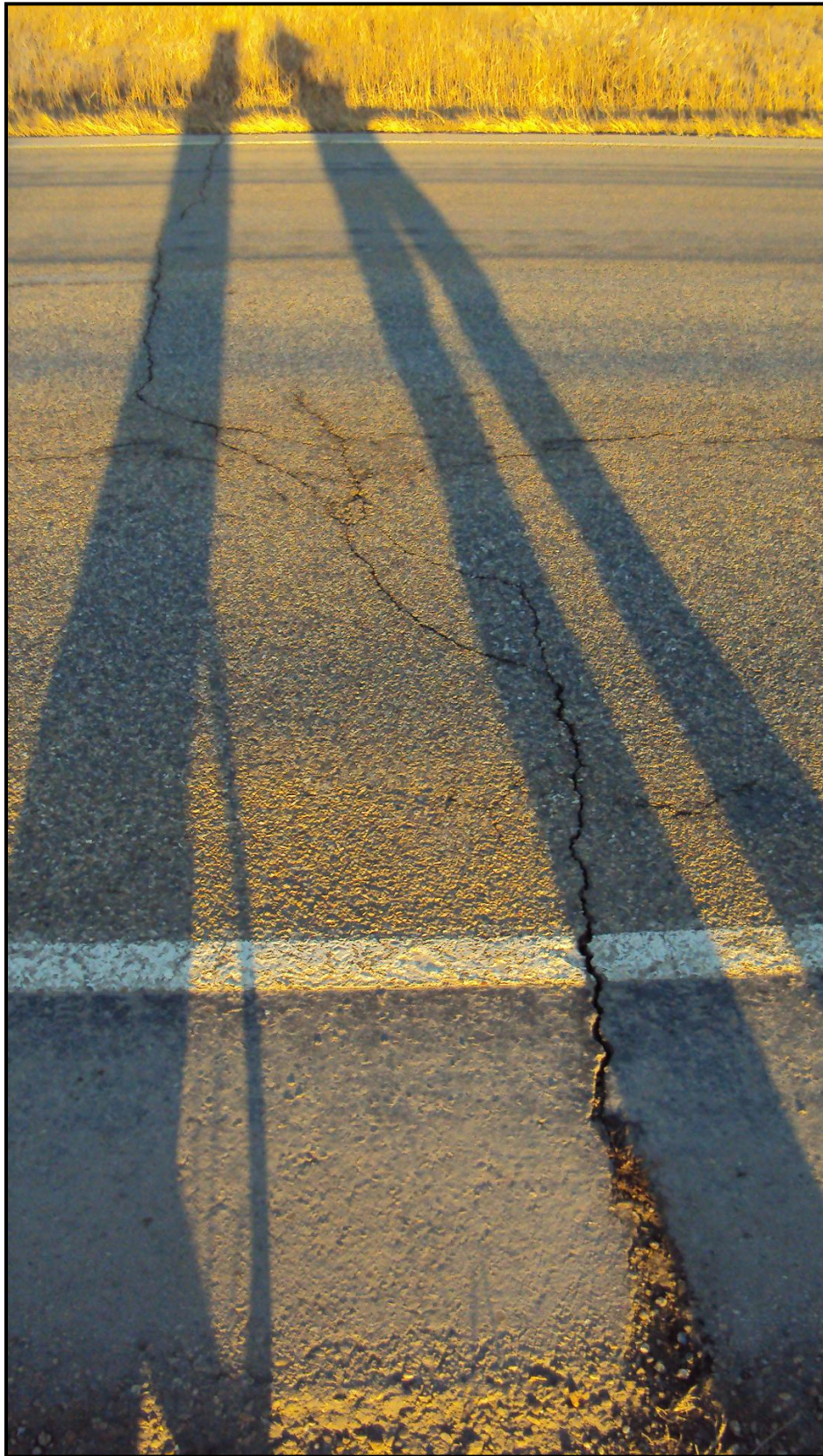
Photo 36. Looking across MT 16 at transverse pavement cracking. Pavement cracking within the travel way measured approximately 0.5 inches in width, approximately every 30 feet. Pavement rutting measured approximately 0.5 inches in depth. RP 19.3.
