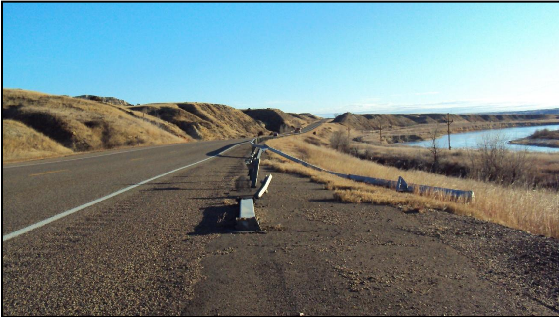
Photo 28. Looking north on MT 16 at damaged guardrail. East side slope transitions from 4:1 to 5:1 approximately 23 feet from northbound travel lane. RP 13.6.
