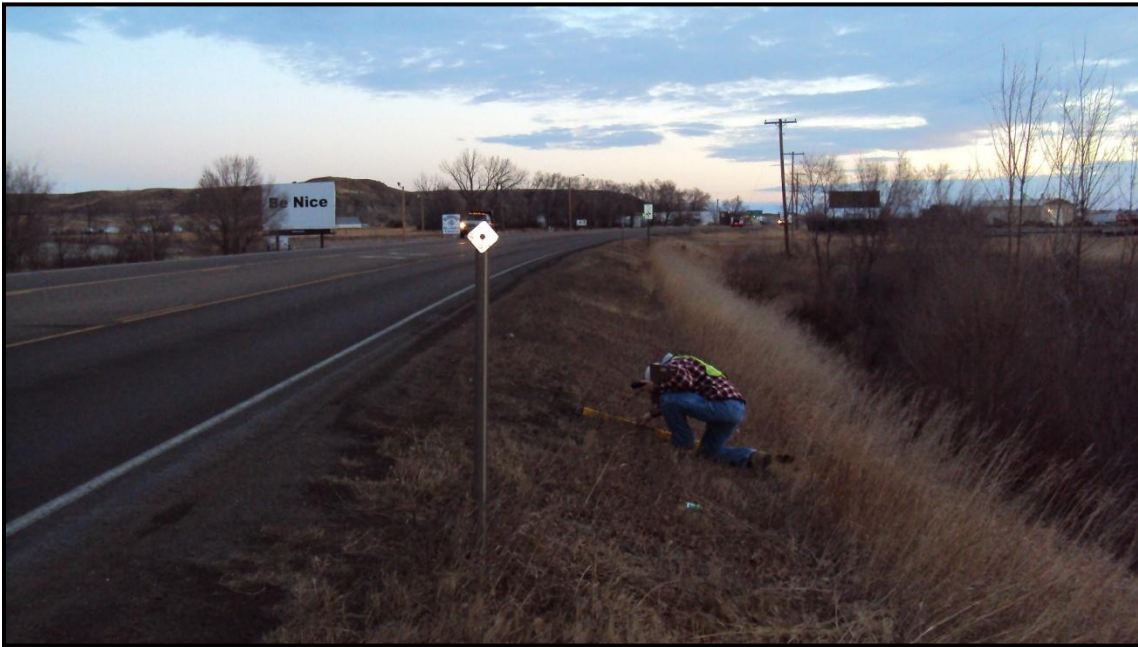
Photo 3. Looking north on MT 16. East side slope transitions from 3:1 to 2:1 approximately 13 feet from northbound travel lane. RP 1.1.
