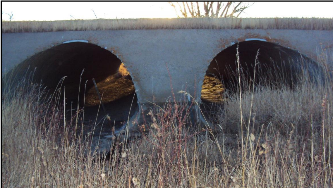
Photo 15. Looking east at 96-inch double arch culverts under MT 16. West side slope was measured at 4:1 to approximately 21 feet from northbound travel lane. RP 7.0.
