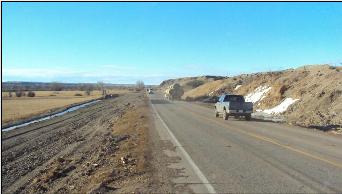
Photo 37. Looking south on MT 16 at narrow shoulder widths, longitudinal pavement cracking, and spot resurfacing. RP 19.6.
