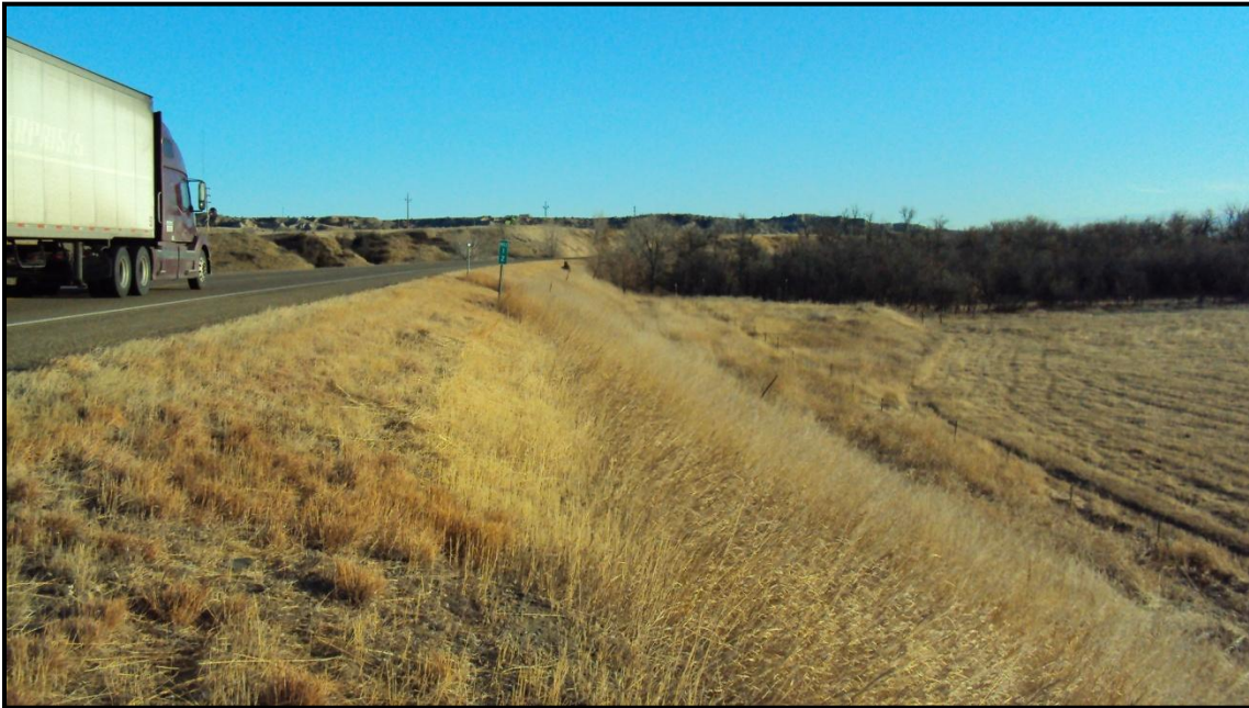
Photo 24. Looking north on MT 16. East side slope transitions from 4:1 to 2:1 approximately 17 feet from northbound travel lane. RP 12.0.
