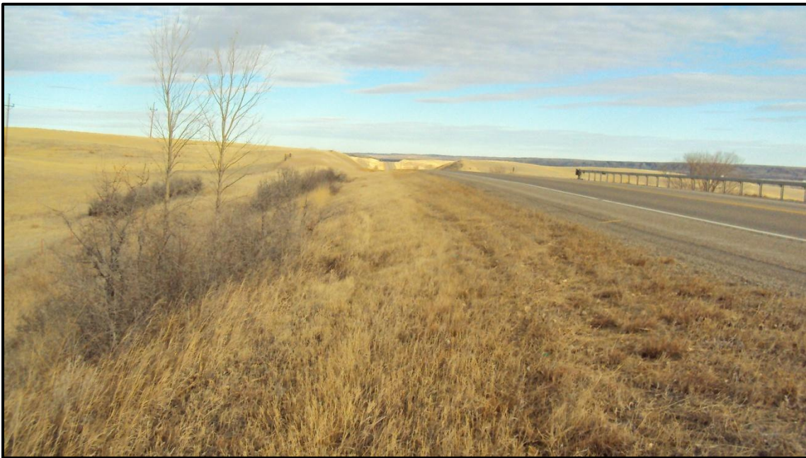
Photo 33. Looking north on MT 16. West side slope transitions from 5:1 to 3:1 approximately 17 feet from southbound travel lane. RP 16.4.
