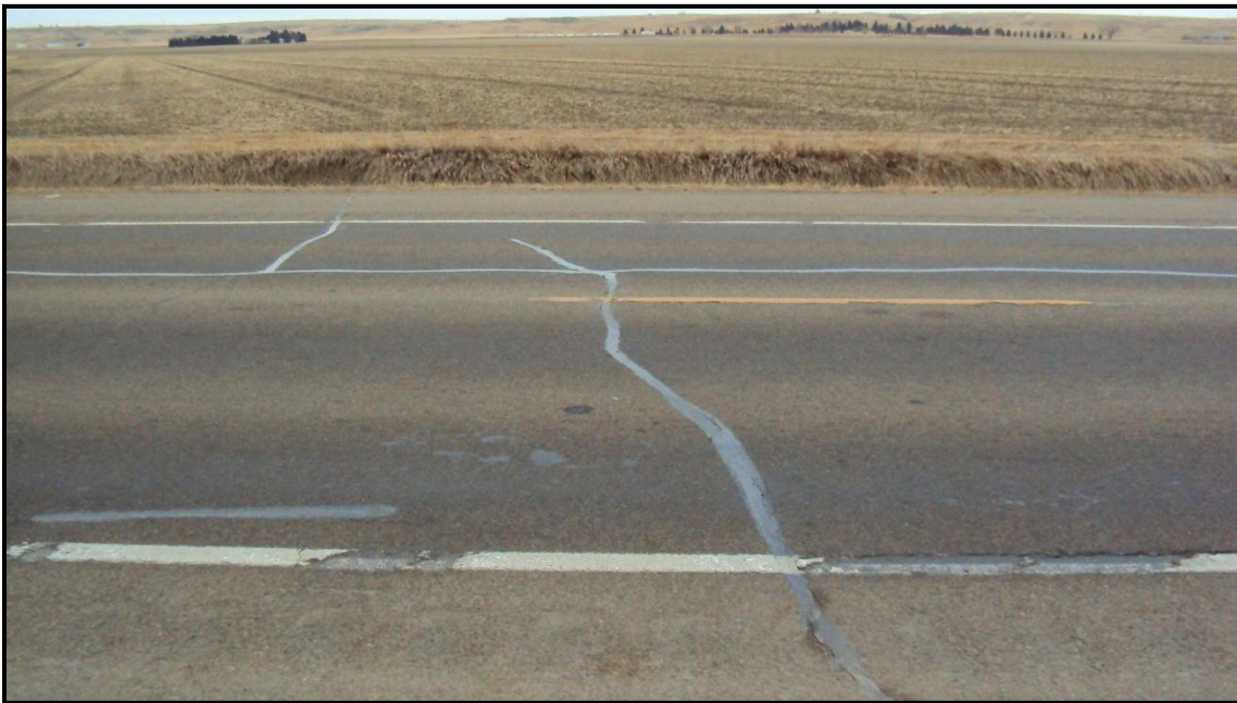
Photo 66. Looking at transverse sealed pavement cracking 0.25 inches in width, approximately every 30 feet. Chip seal peeling was observed on the travel way white line. No measurable pavement rutting was observed within the travel way. RP 54.0.
