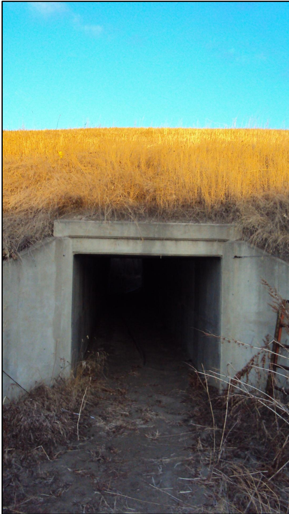
Photo 8. Looking west at a box culvert/wildlife underpass under MT 16. East side slope transitions from 4:1 to 2:1 approximately 18 feet from northbound travel lane. RP 2.4.
