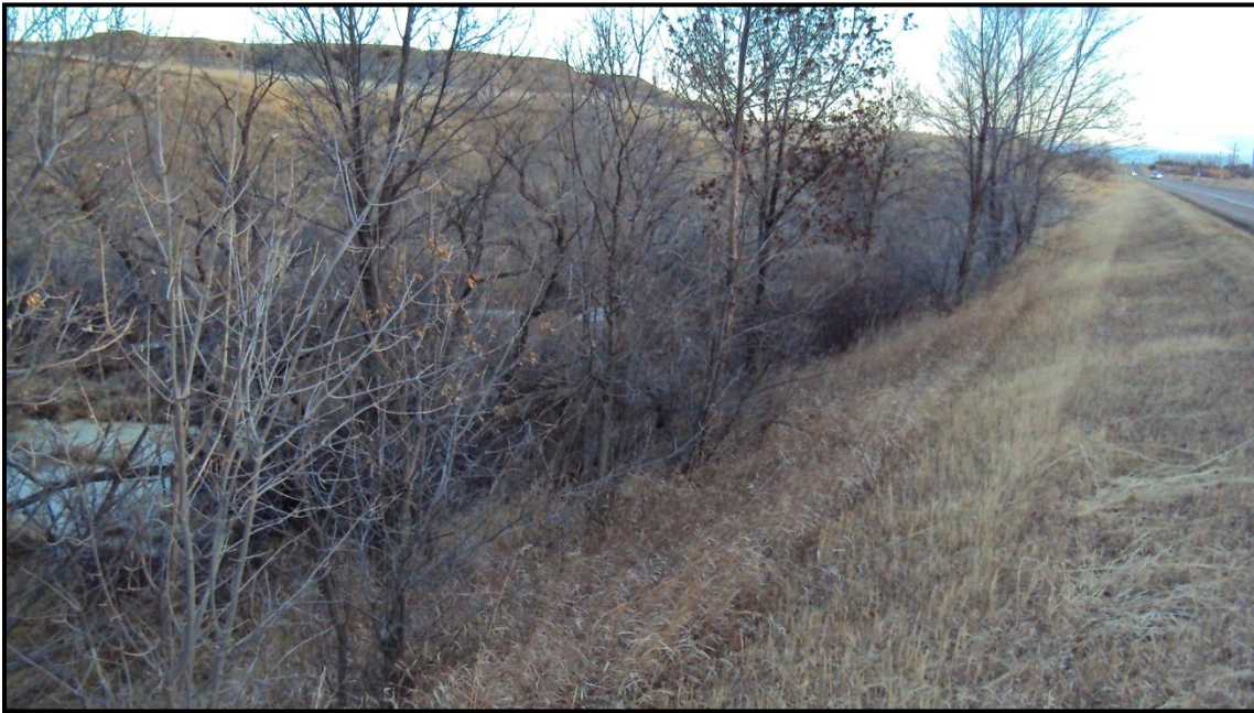
Photo 7. Looking north on the west side slope of MT 16. West side slope transitions from 4:1 to 2:1 approximately 20 feet from southbound travel lane. Areas exhibiting wetland characteristics observed west of MT 16. RP 1.7.
