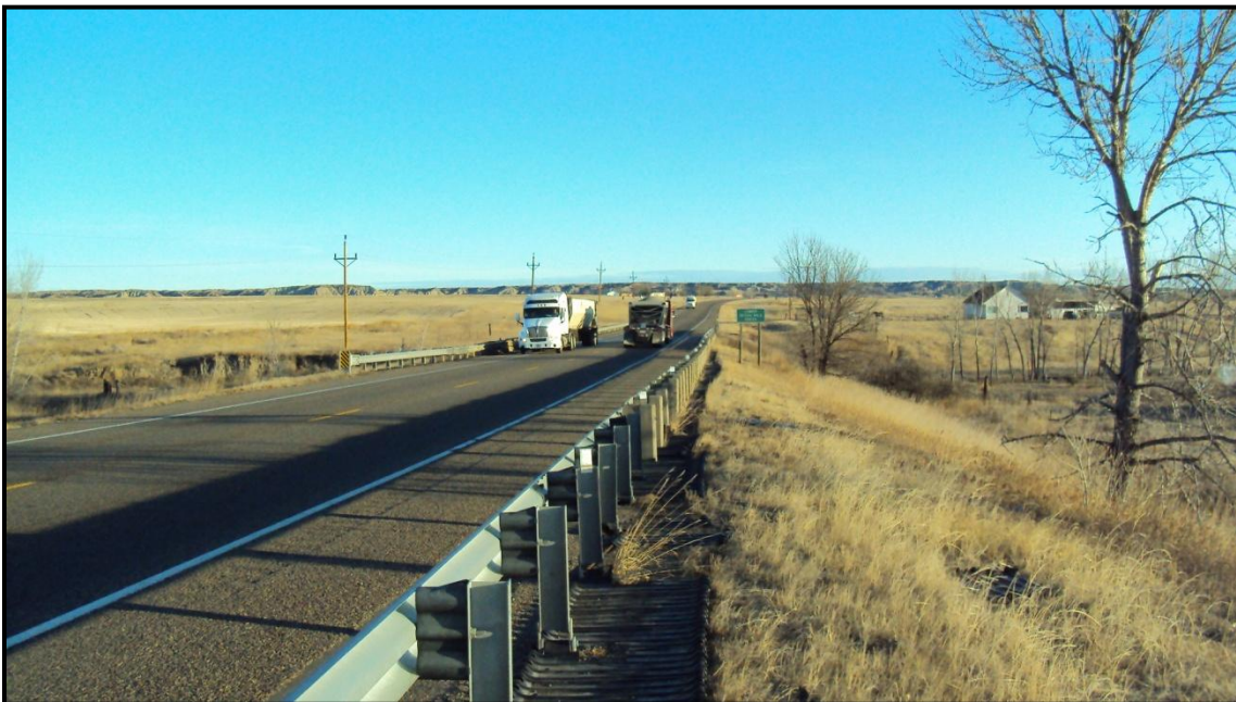
Photo 20. Looking south on MT 16 at Lower Seven Mile Creek. East side slope transitions from 4:1 to 2:1 approximately 15 feet from the northbound travel lane. RP 10.1.
