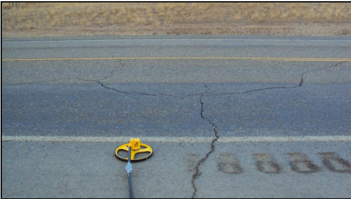
Photo 46. Looking across MT 16 at continuous transverse pavement cracking. Pavement cracking within the travel way measured approximately 0.5 inches in width, approximately every 35 feet. RP 29.0.
