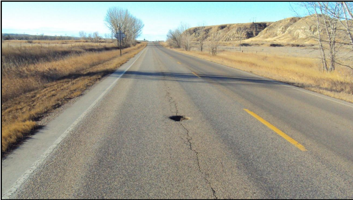
Photo 35. Looking south on MT 16 at longitudinal pavement cracking and pothole. RP 19.3.
