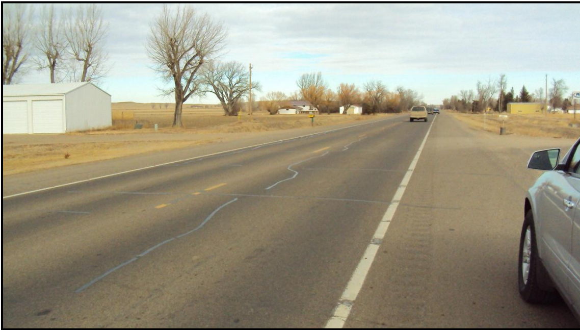
Photo 67. Looking north on MT 200 at transverse and longitudinal pavement crack sealing. RP 56.0.
