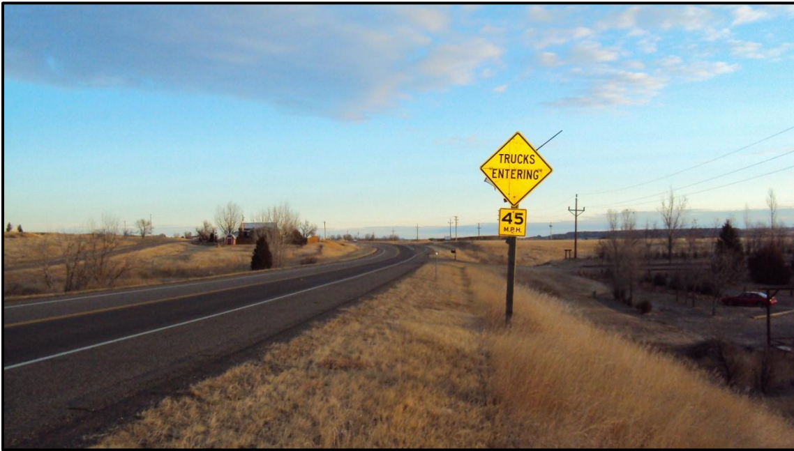
Photo 9. Looking north on MT 16 at trucks entering 45 mph advisory sign. East side slope transitions from 5:1 to 2:1 approximately 18 feet from northbound travel lane. RP 2.8.
