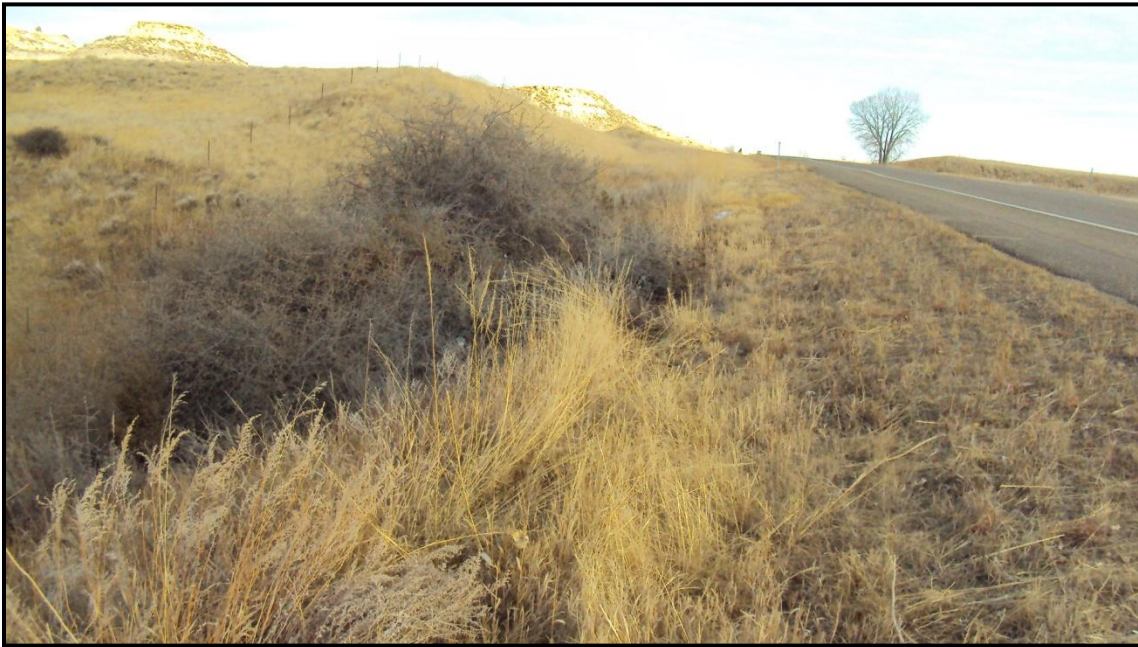
Photo 30. Looking south on MT 16. West side slope transitions from 4:1 to 2:1 approximately 20 feet from northbound travel lane. RP 14.4.
