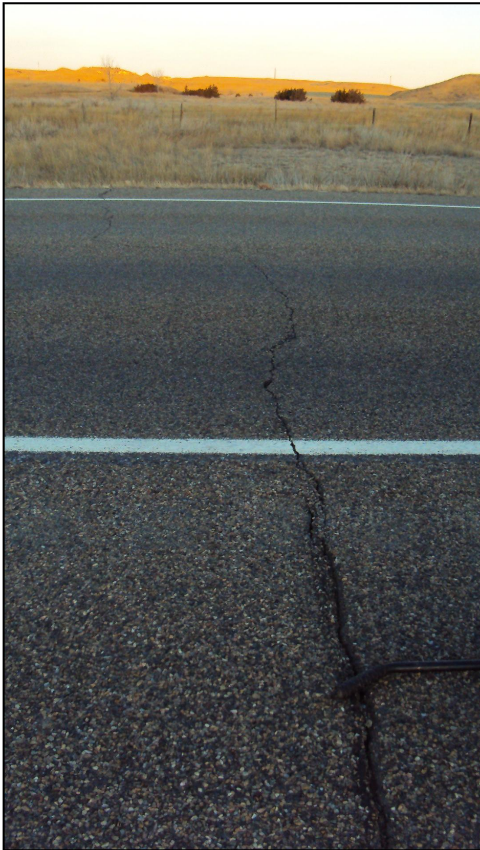
Photo 16. Looking across MT 16 at transverse pavement cracking. Pavement cracking within the travel way measured approximately 0.125 inches, approximately every 50 feet. Pavement rutting measured at approximately 0.5 centimeters. RP 8.3.
