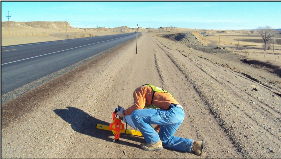
Photo 41. Looking north on MT 16. East side slope transitions from 5:1 to 3:1 approximately 28 feet from northbound travel lane. RP 22.5.
