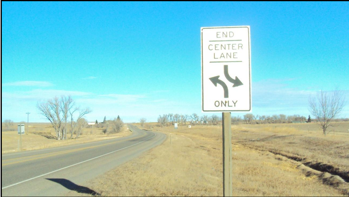
Photo 51. Looking north on MT 16 at end of two-way left-turn lane and restored posted speed limits (60 mph for trucks, 70 mph for vehicles). RP 32.3.
