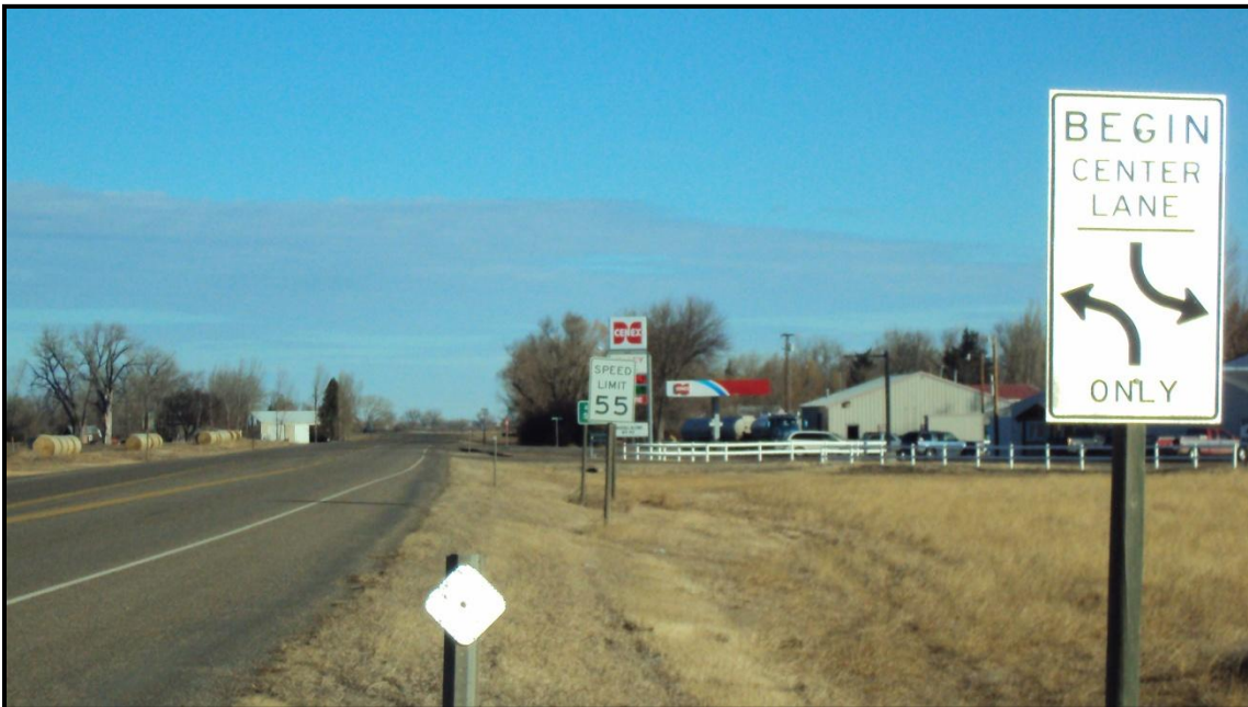
Photo 50. Looking north on MT 16 at beginning of two-way left-turn lane and reduced posted speed limit (55 mph for all vehicles) through Savage, MT. RP 31.5.
