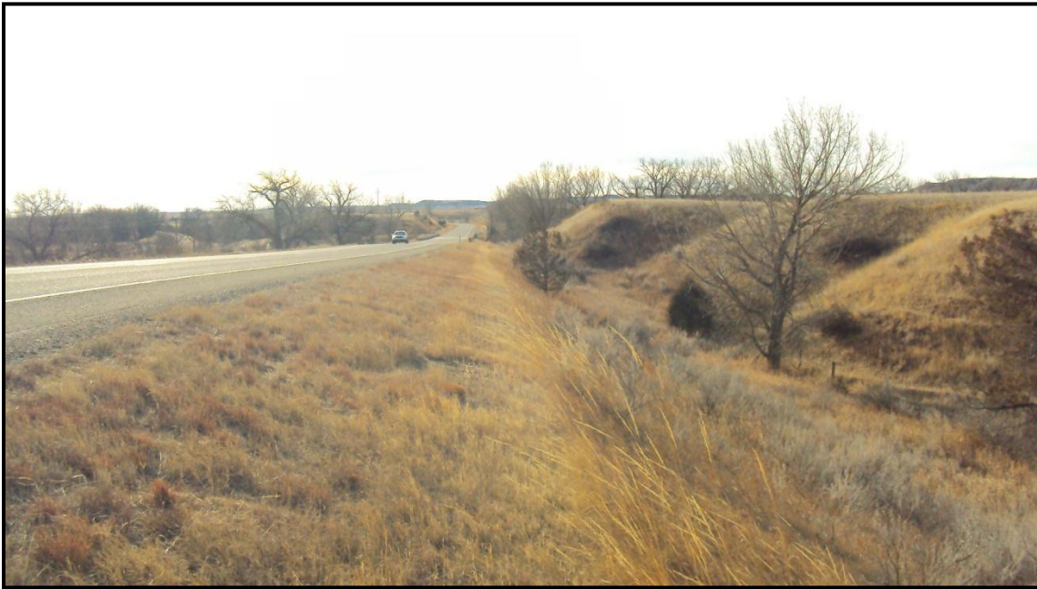
Photo 27. Looking north on MT 16. East side slope transitions from 4:1 to 2:1 approximately 20 feet from northbound travel lane. RP 12.7.
