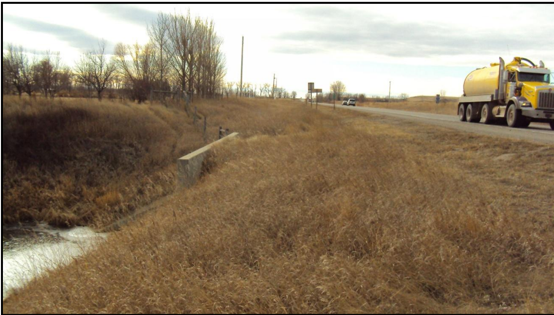
Photo 72. Looking south on MT 200 at Second Hay Creek. Distance from the northbound travel lane to concrete wall is approximately 40 feet. RP 60.1
