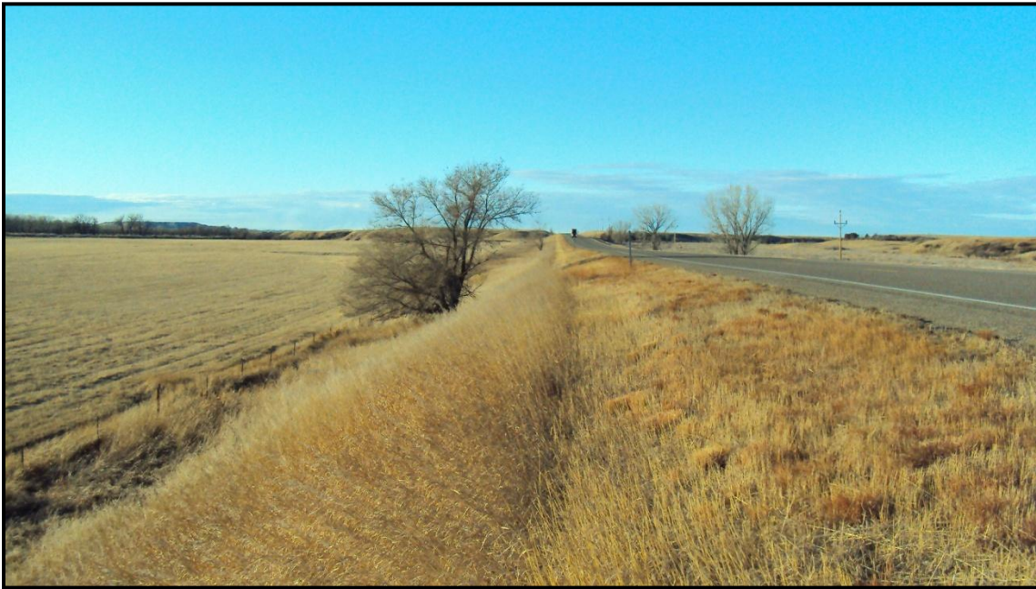
Photo 23. Looking south on MT 16. West side slope transitions from 4:1 to 2:1 approximately 17 feet from southbound travel lane. RP 12.0.
