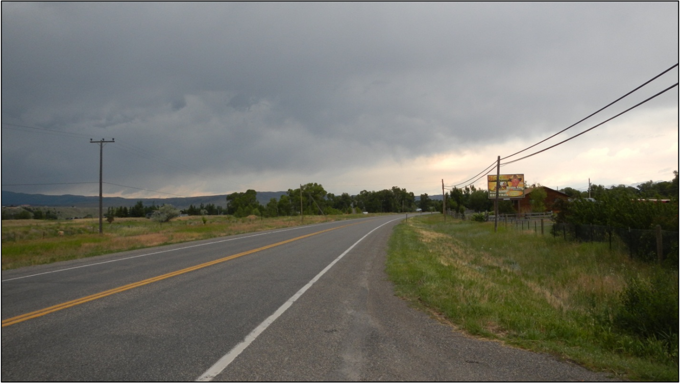
PHOTO 62: RP 51.0, LOOKING NORTH
