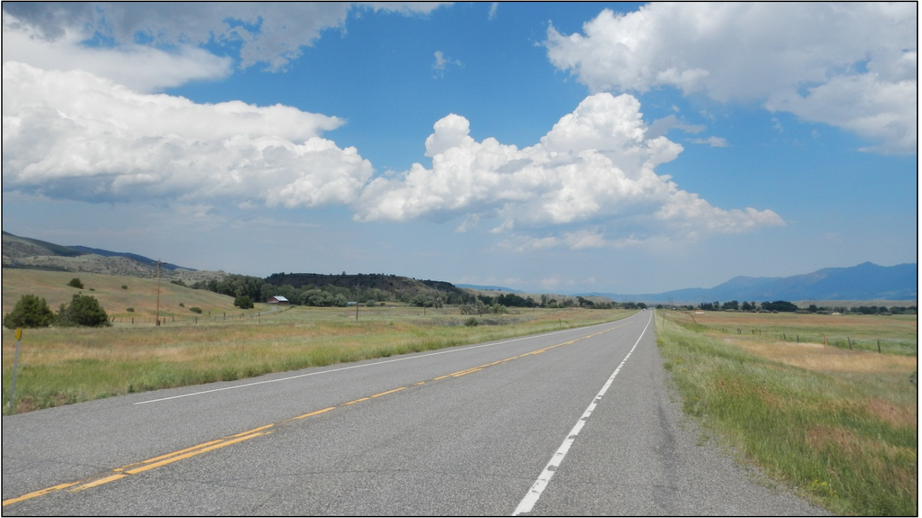
PHOTO 40: RP 29.3, LOOKING NORTHEAST
