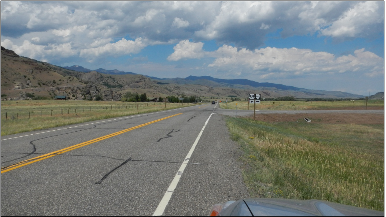
PHOTO 29: RP 19.9, LOOKING NORTH (NOTE INTERSECTION WITH S-540)
