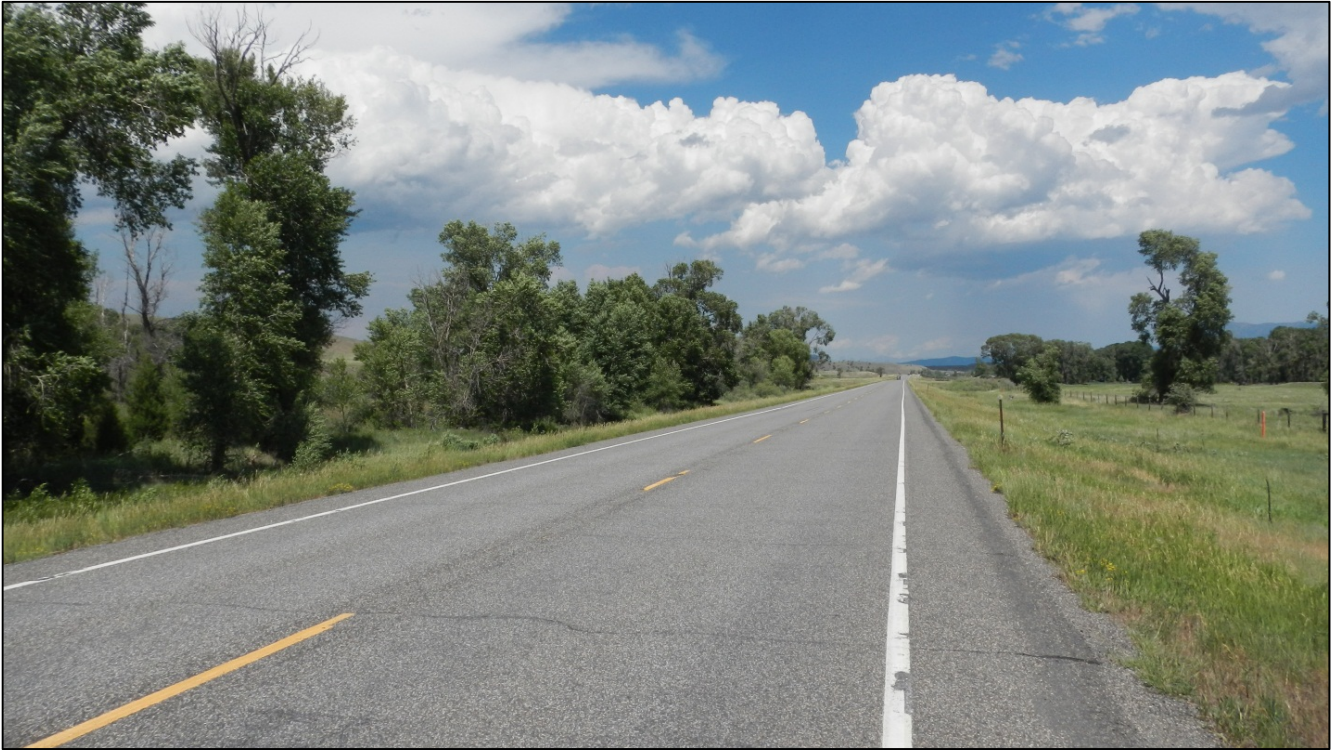
PHOTO 44: RP 32.9, LOOKING NORTHEAST
