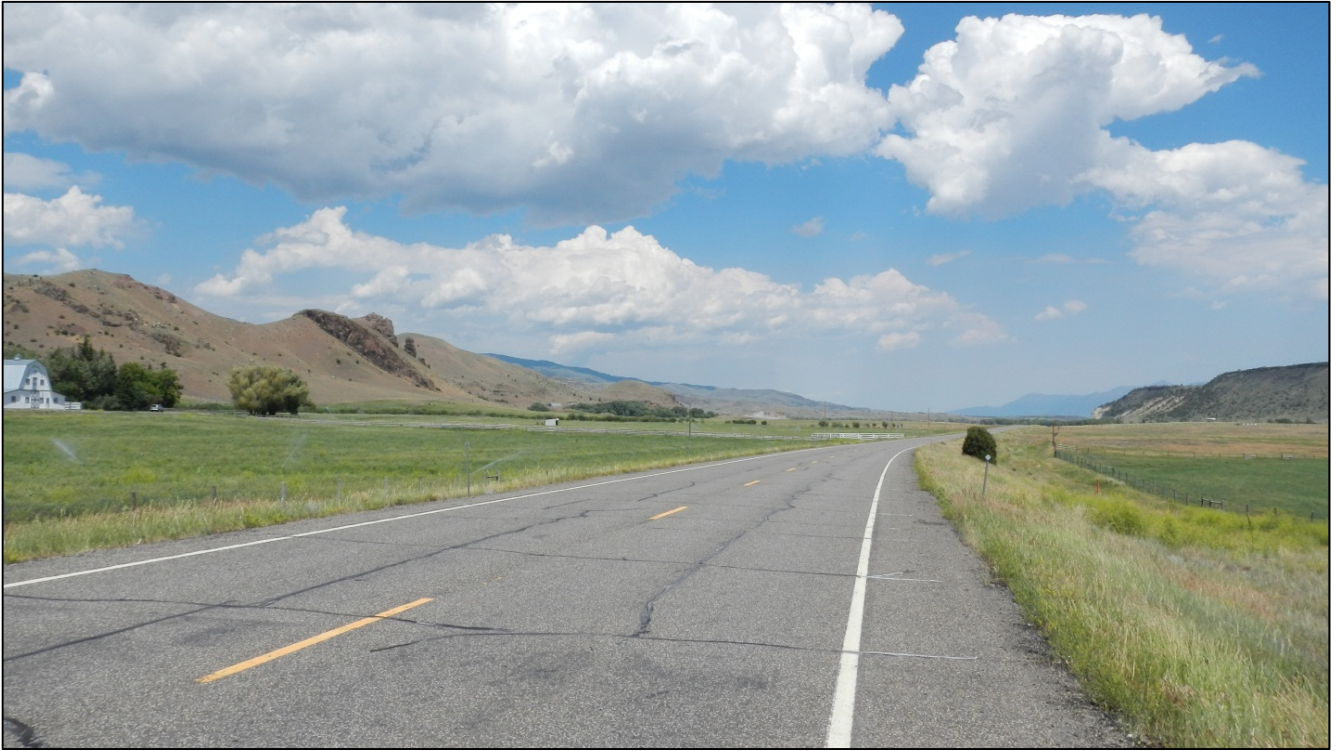
PHOTO 32: RP 22.0, LOOKING NORTHEAST
