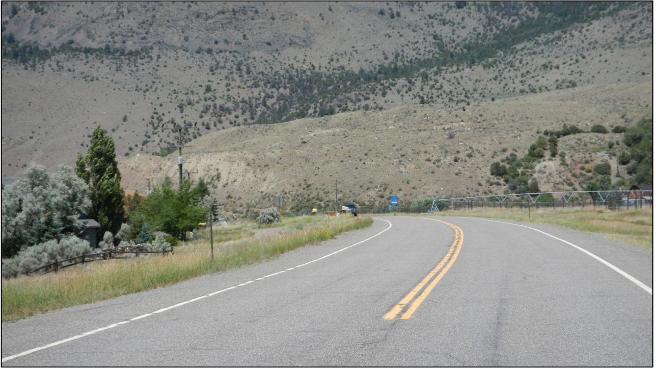
PHOTO 15: RP 10.8, LOOKING NORTHWEST
