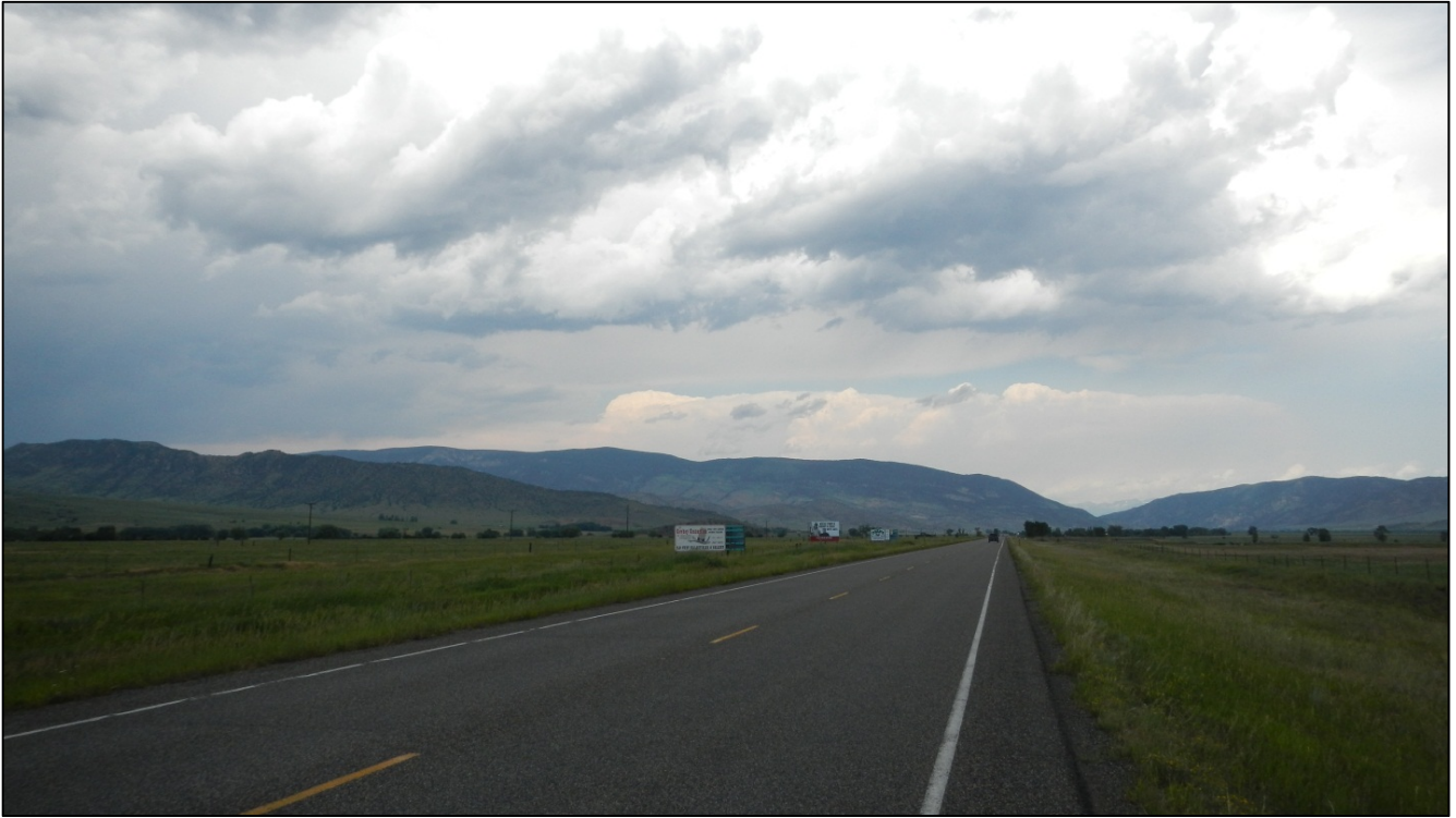
PHOTO 52: RP 40.9, LOOKING NORTH
