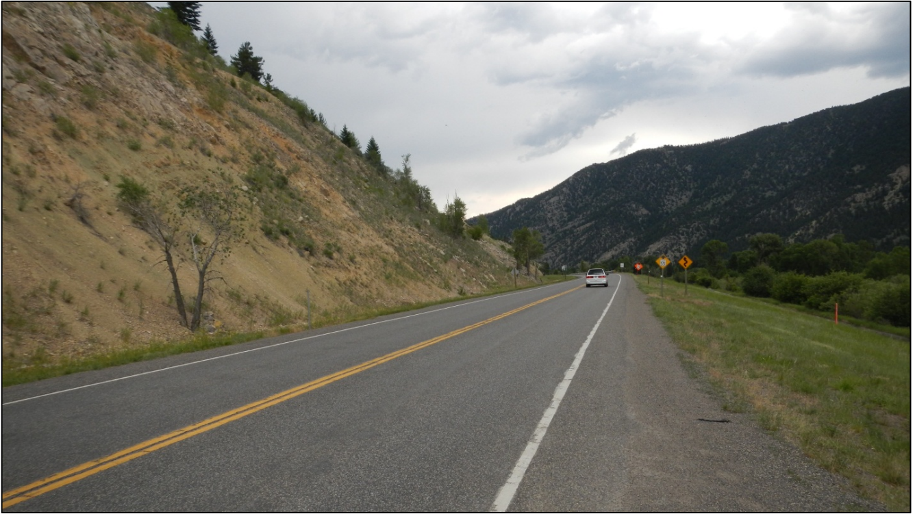
PHOTO 60: RP 48.9, LOOKING NORTHEAST
