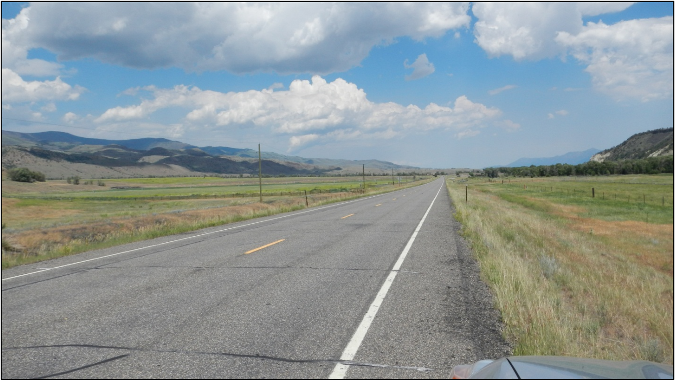
PHOTO 33: RP 23.0, LOOKING NORTHEAST
