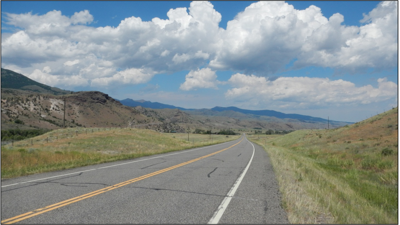
PHOTO 28: RP 19.5, LOOKING NORTH
