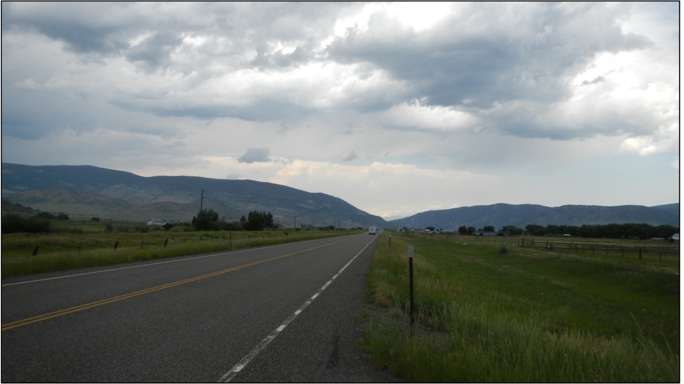
PHOTO 54: RP 42.8, LOOKING NORTH
