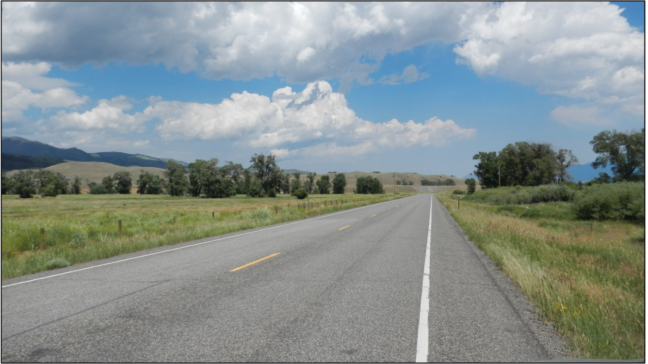
PHOTO 36: RP 25.0, LOOKING NORTHEAST
