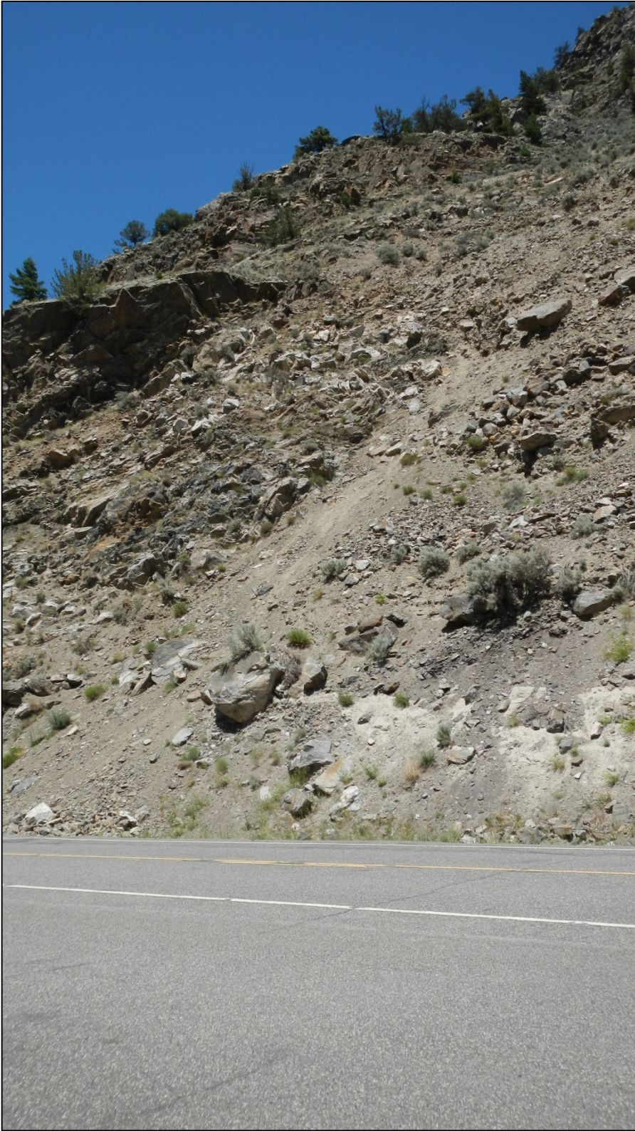
PHOTO 21: RP 13.5, LOOKING WEST (NOTE ROCKFALL ON RIGHT)
