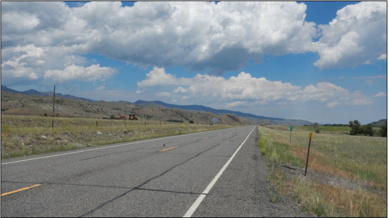
PHOTO 31: RP 20.9, LOOKING NORTHEAST
