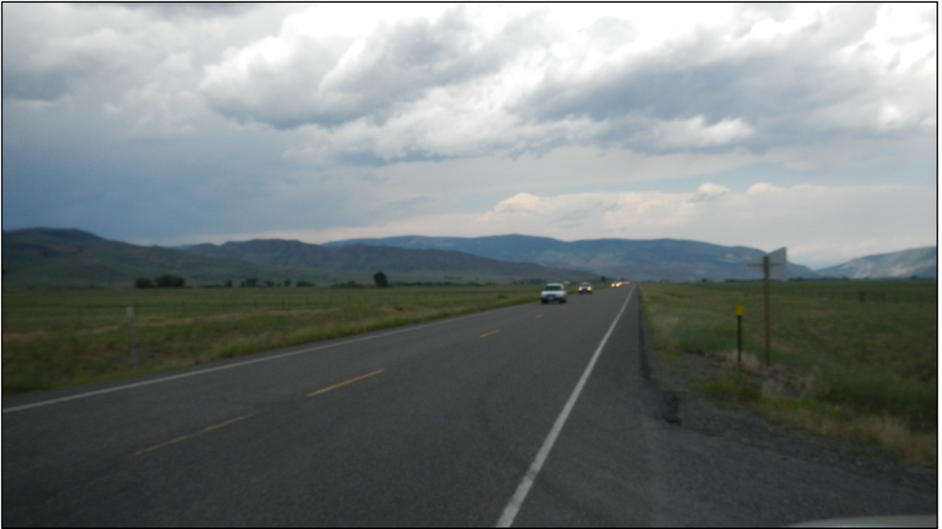
PHOTO 51: RP 40.0, LOOKING NORTH
