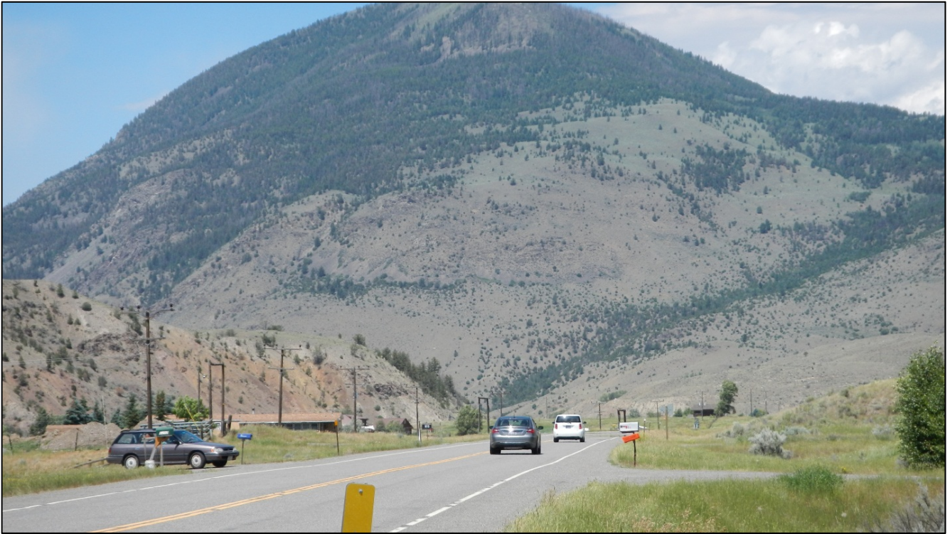
PHOTO 14: RP 10.0, LOOKING NORTHWEST
