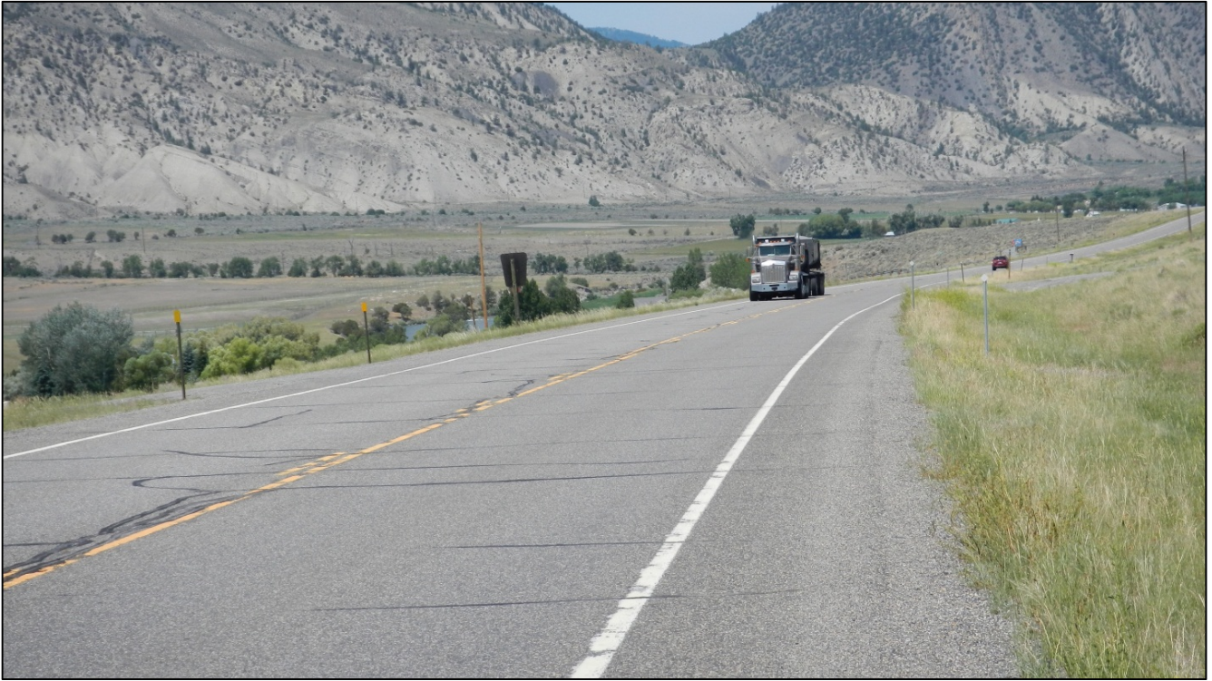
PHOTO 7: RP 3.1, LOOKING NORTHWEST
