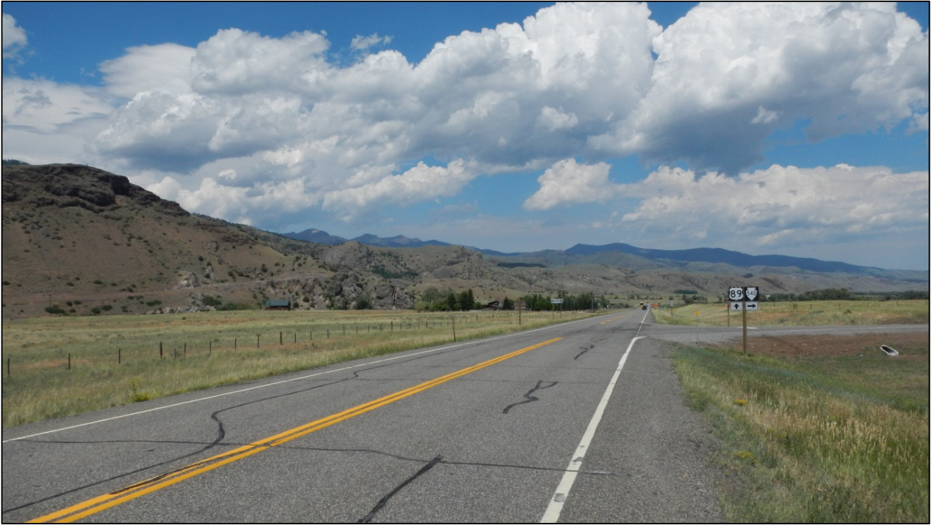
PHOTO 30: RP 19.9, LOOKING NORTH (NOTE INTERSECTION WITH S-540)
