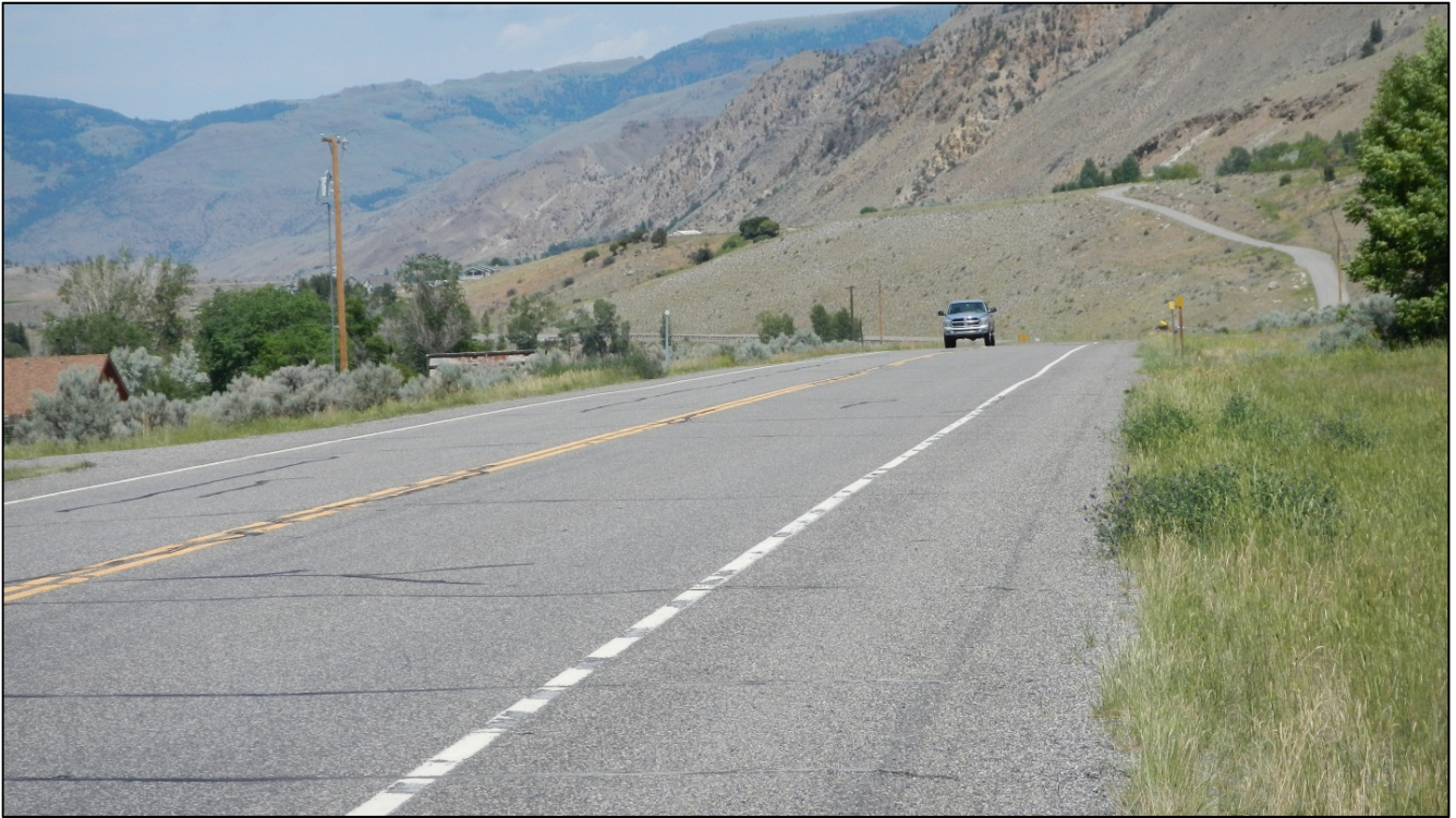
PHOTO 8: RP 4.3, LOOKING NORTH
