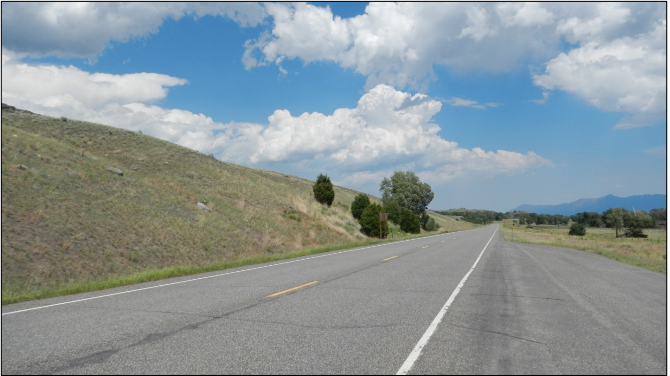
PHOTO 39: RP 28.0, LOOKING NORTHEAST
