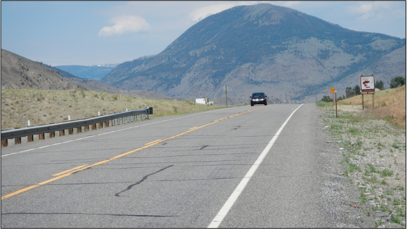
PHOTO 11: RP 6.8, LOOKING NORTHWEST
