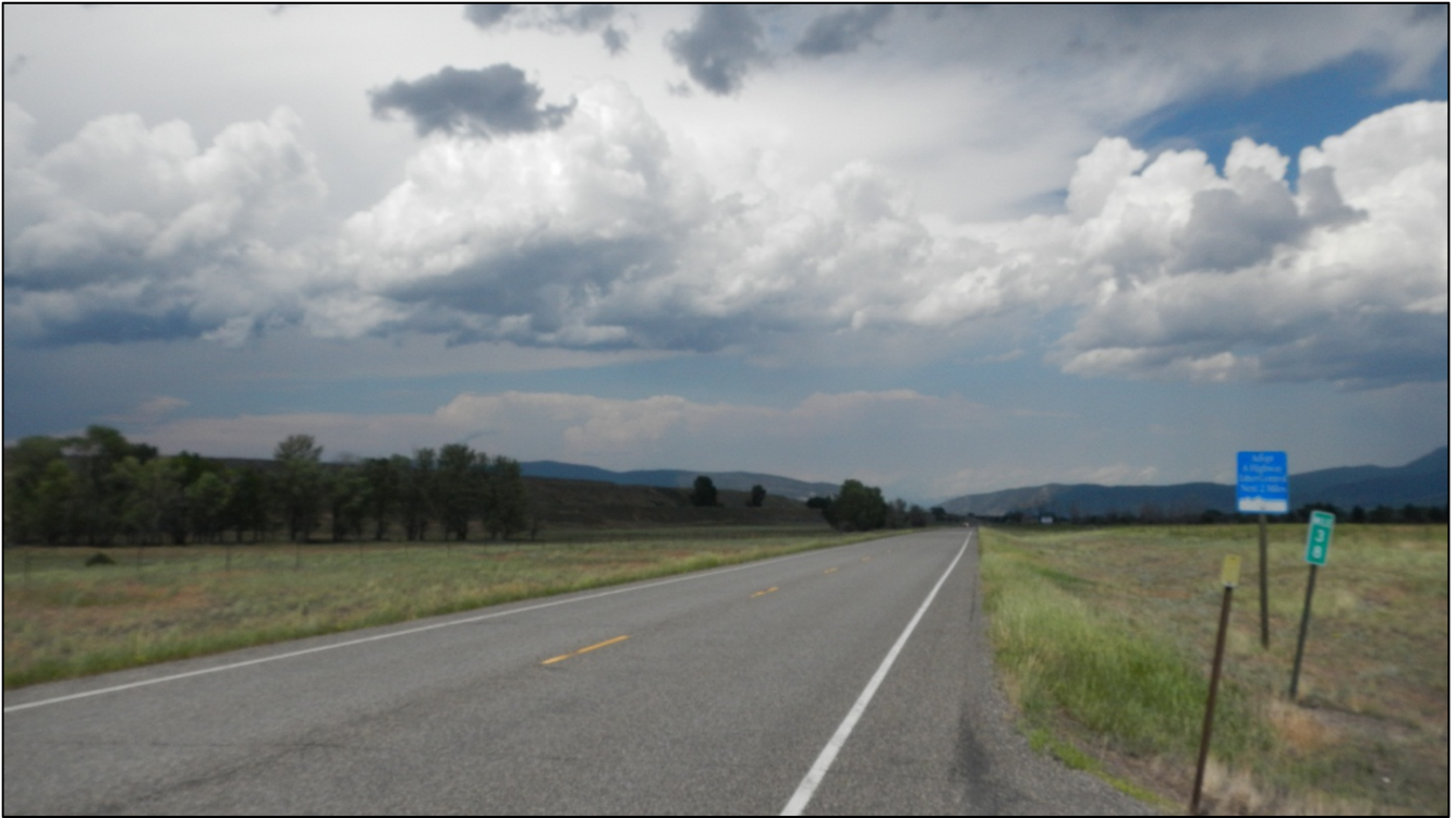
PHOTO 49: RP 37.9, LOOKING NORTH
