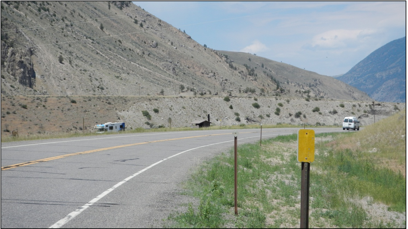
PHOTO 10: RP 6.0, LOOKING NORTH
