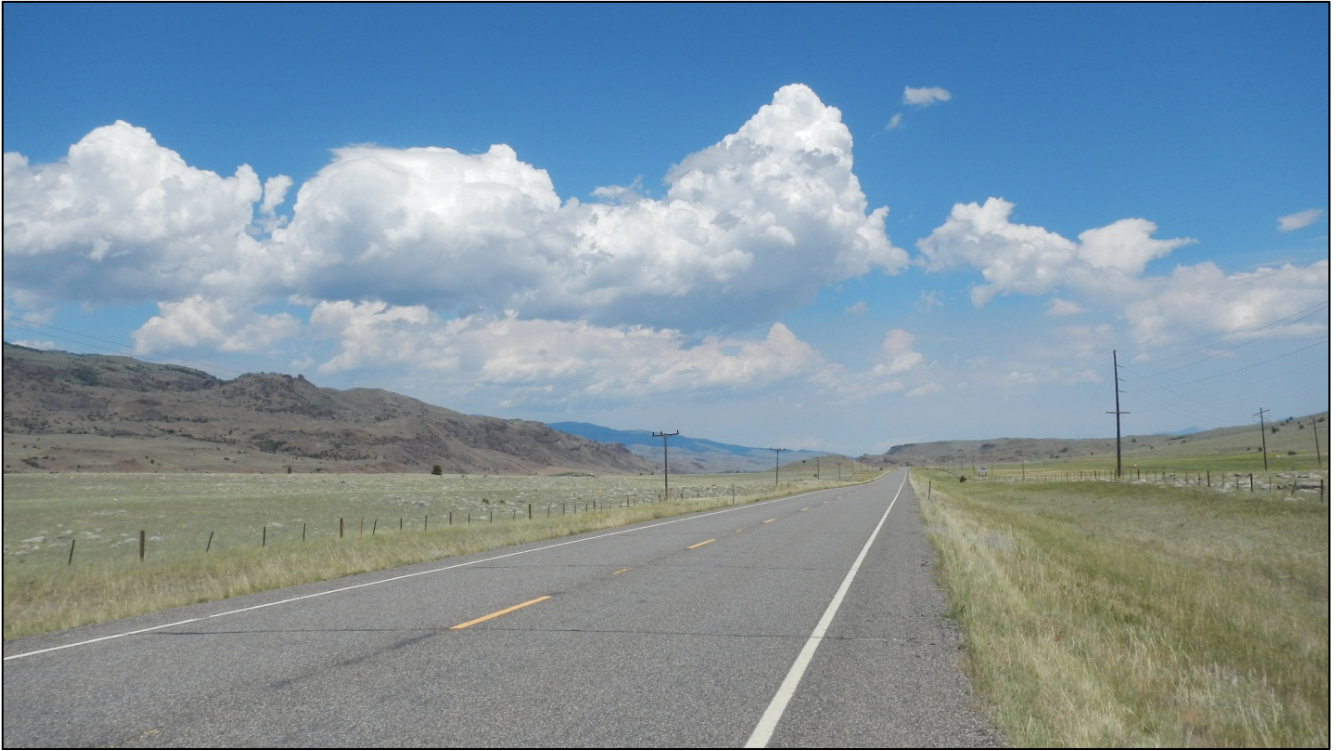
PHOTO 26: RP 17.0, LOOKING NORTHEAST
