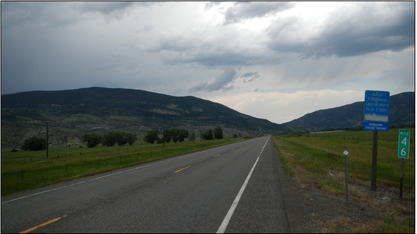
PHOTO 57: RP 46.0, LOOKING NORTHEAST
