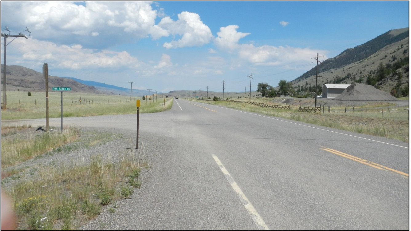
PHOTO 25: RP 16.6, LOOKING NORTHEAST (NOTE PUBLIC ROAD INTERSECTION)
