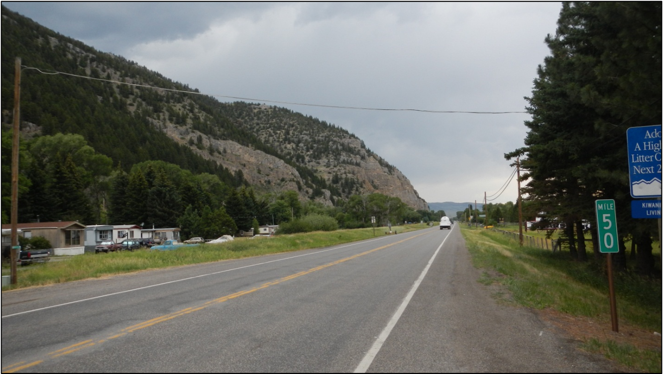
PHOTO 61: RP 50.0, LOOKING NORTH
