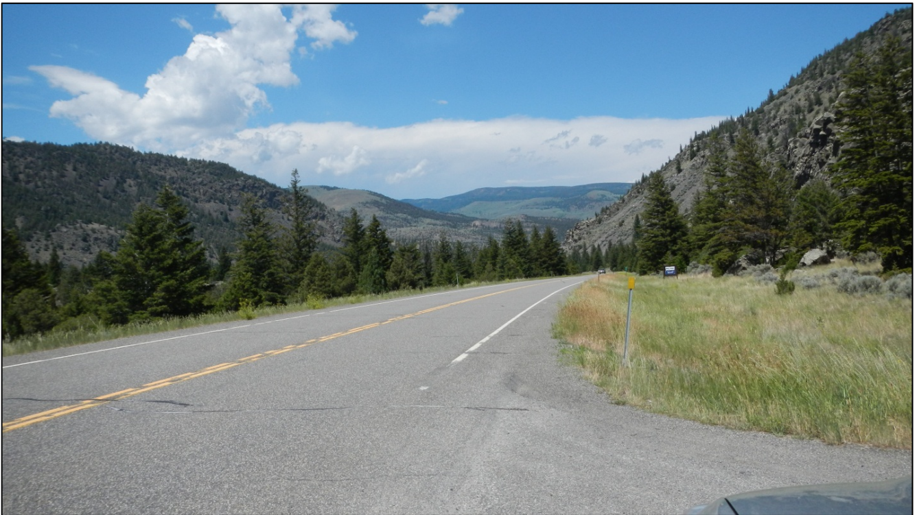
PHOTO 23: RP 14.9, LOOKING WEST
