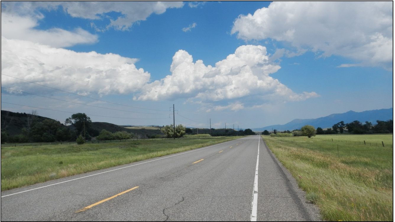
PHOTO 41: RP 29.9, LOOKING NORTHEAST
