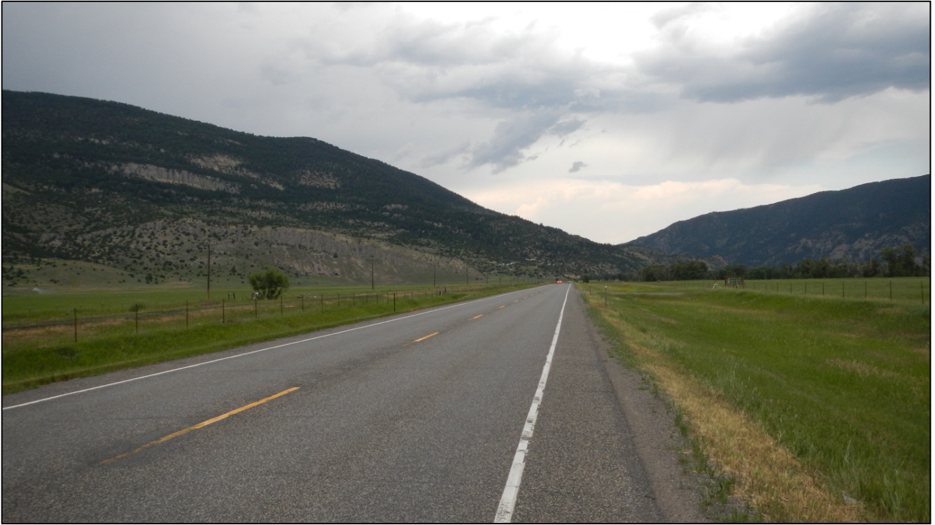
PHOTO 58: RP 46.9, LOOKING NORTHEAST
