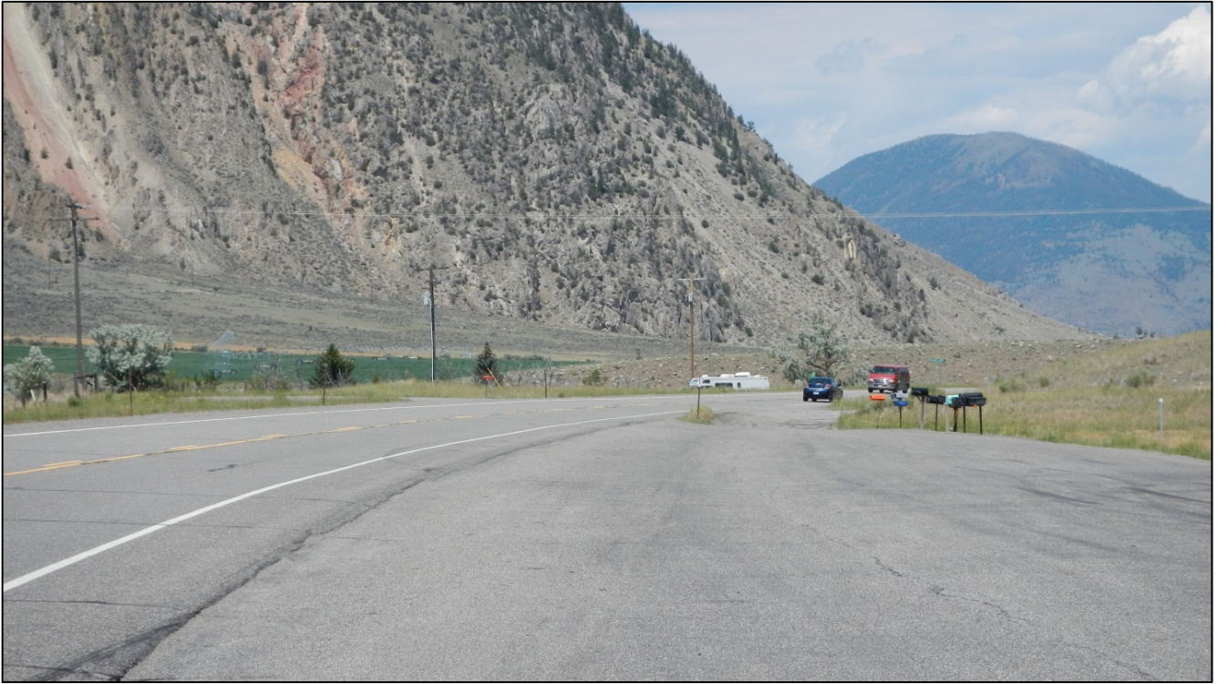
PHOTO 9: RP 5.2, LOOKING NORTHWEST
