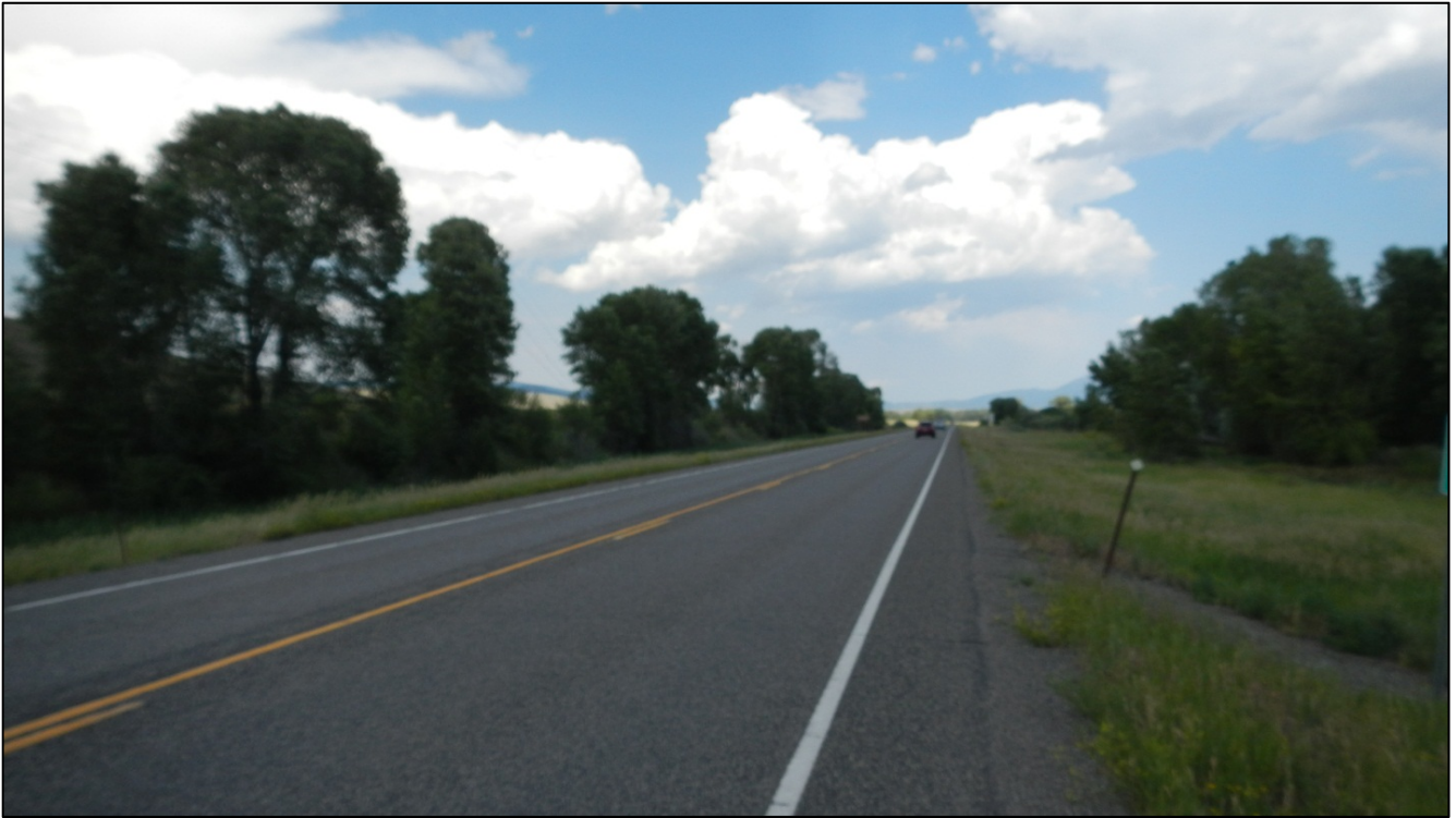
PHOTO 43: RP 31.9, LOOKING NORTHEAST
