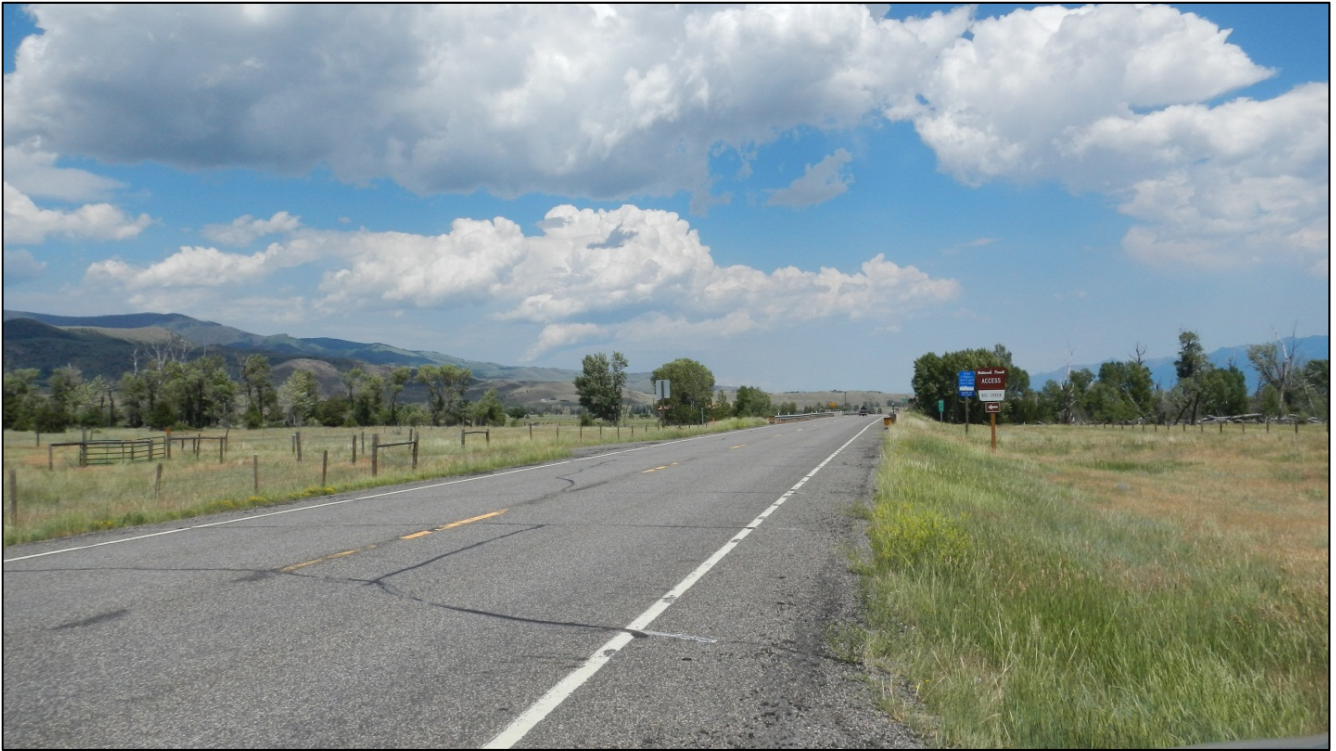
PHOTO 35: RP 23.9, LOOKING NORTHEAST
