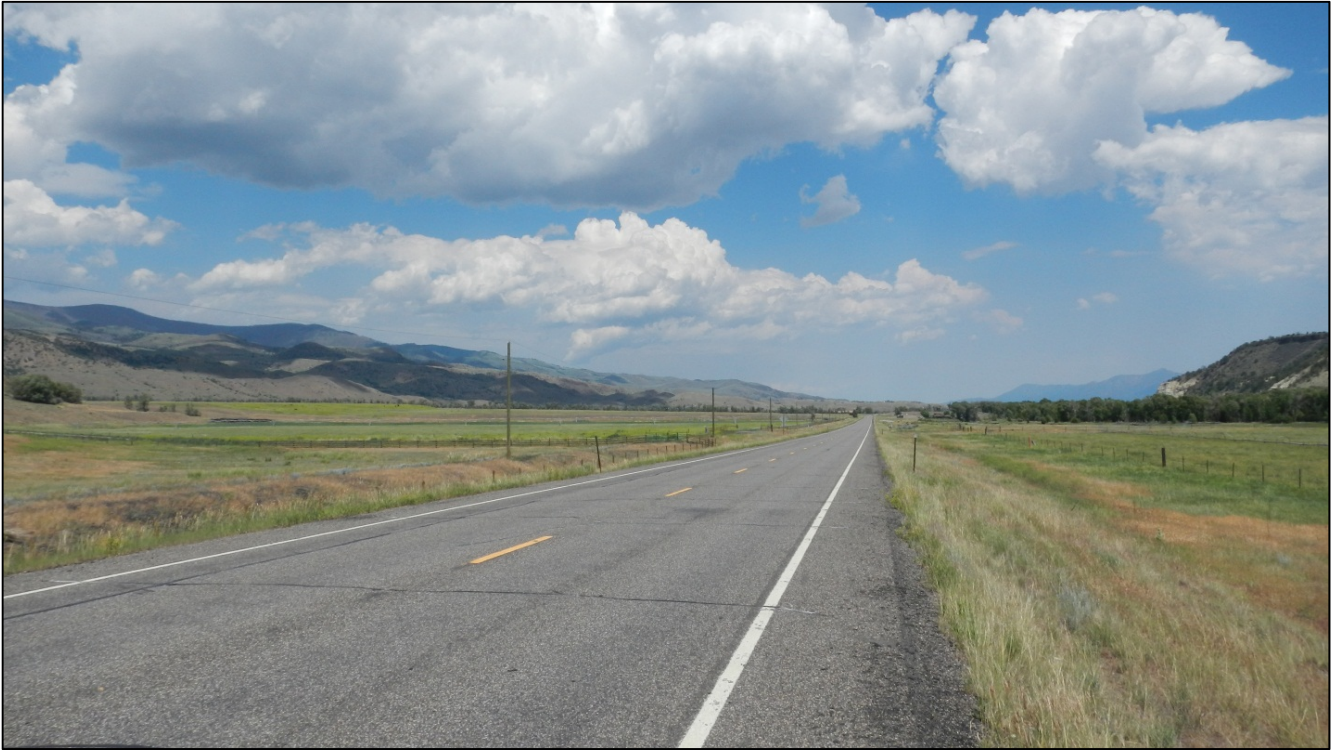
PHOTO 34: RP 23.0, LOOKING NORTHEAST
