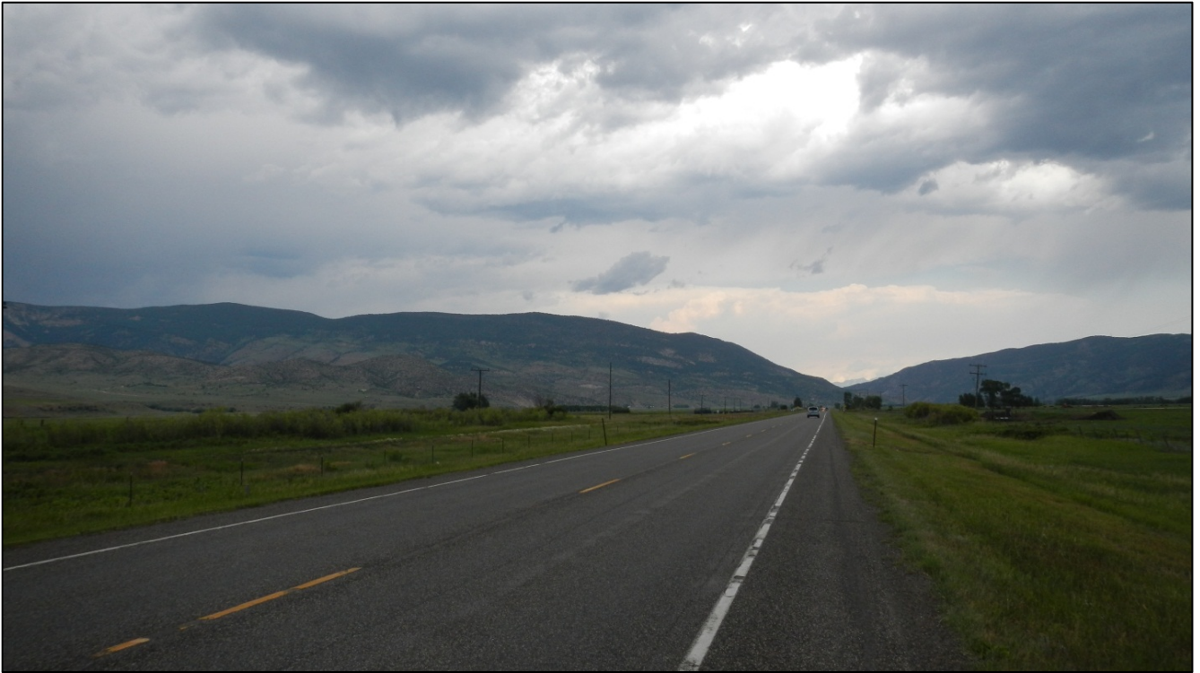
PHOTO 55: RP 43.9, LOOKING NORTH
