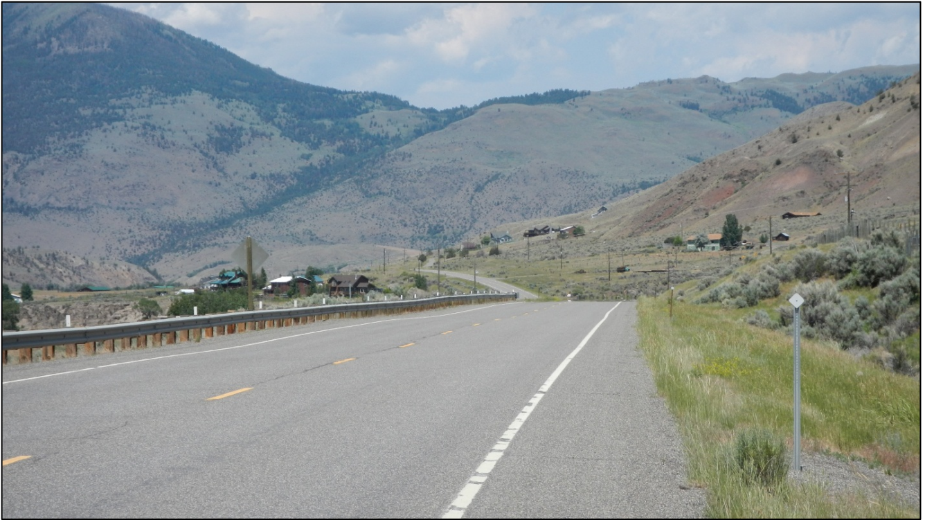
PHOTO 12: RP 8.0, LOOKING NORTH
