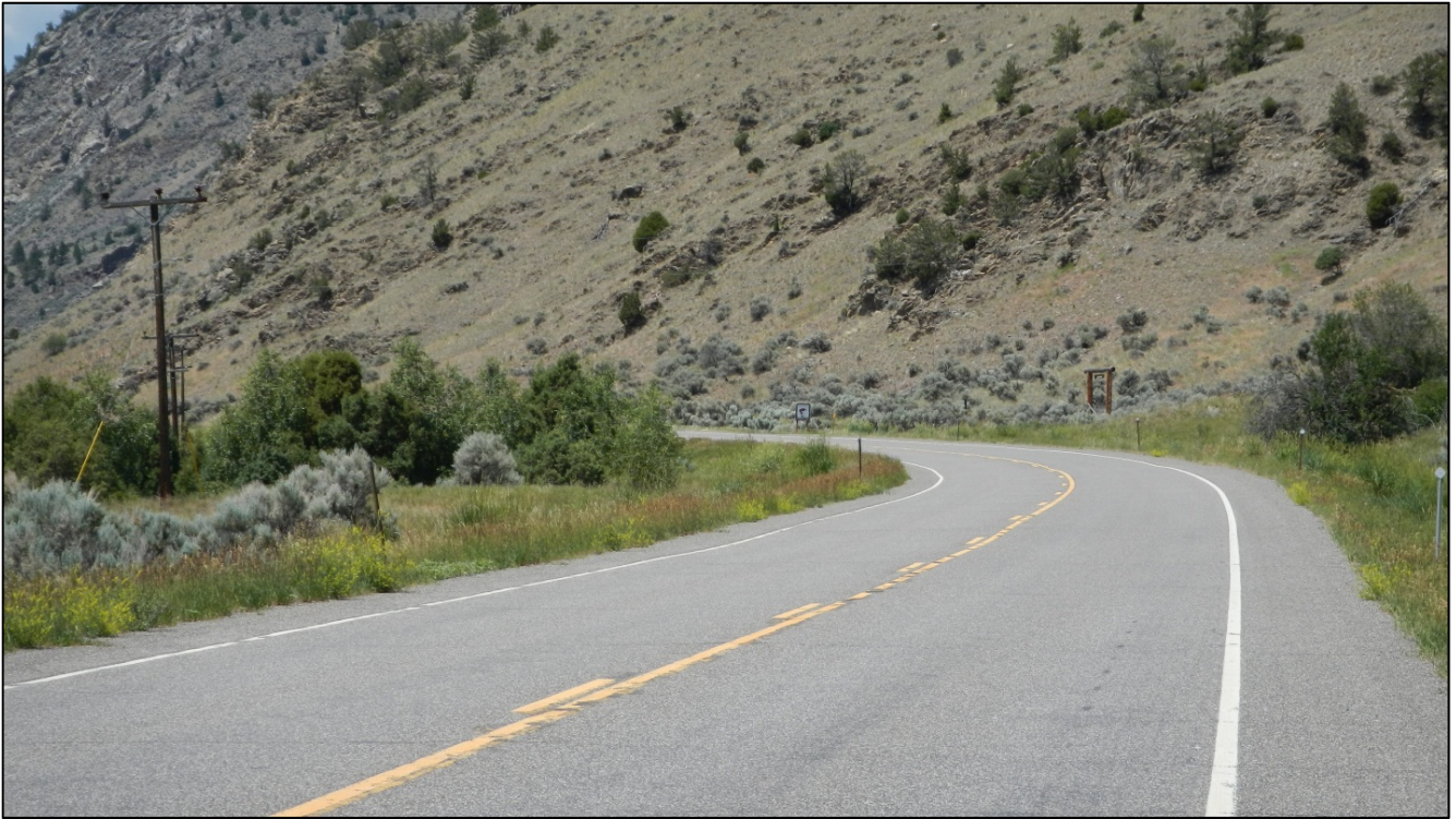
PHOTO 16: RP 12.0, LOOKING WEST
