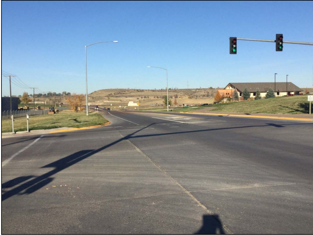
Photo 31: Looking west from the intersection with 38 th Street North (RP 5.4)
