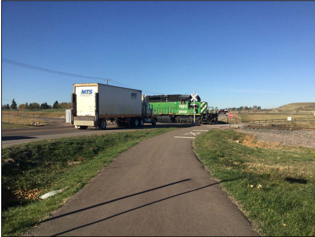
Photo 30: Looking west at the railroad crossing (RP 5.3)
