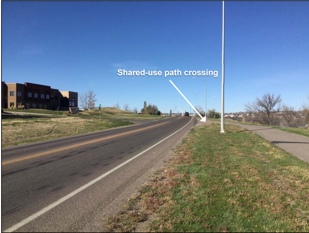
Photo 4: Looking west near the intersection with 19 th Street North (RP 3.8)
