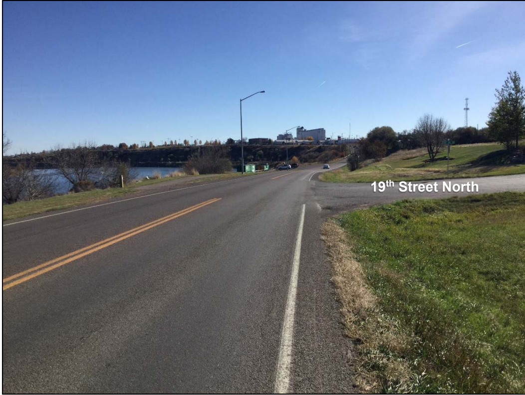
Photo 3: Looking east at the intersection with 19 th Street North (RP 3.7)
