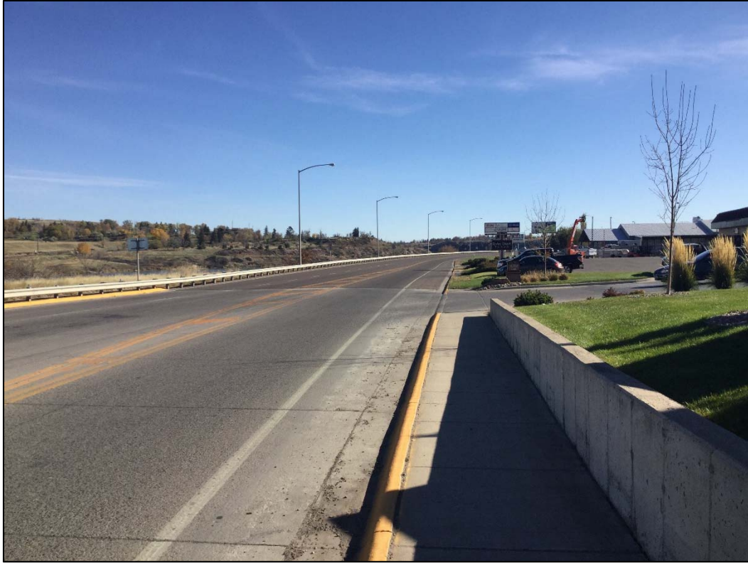
Photo 1: Looking east near the intersection with 15 th Street North (RP 3.5)
