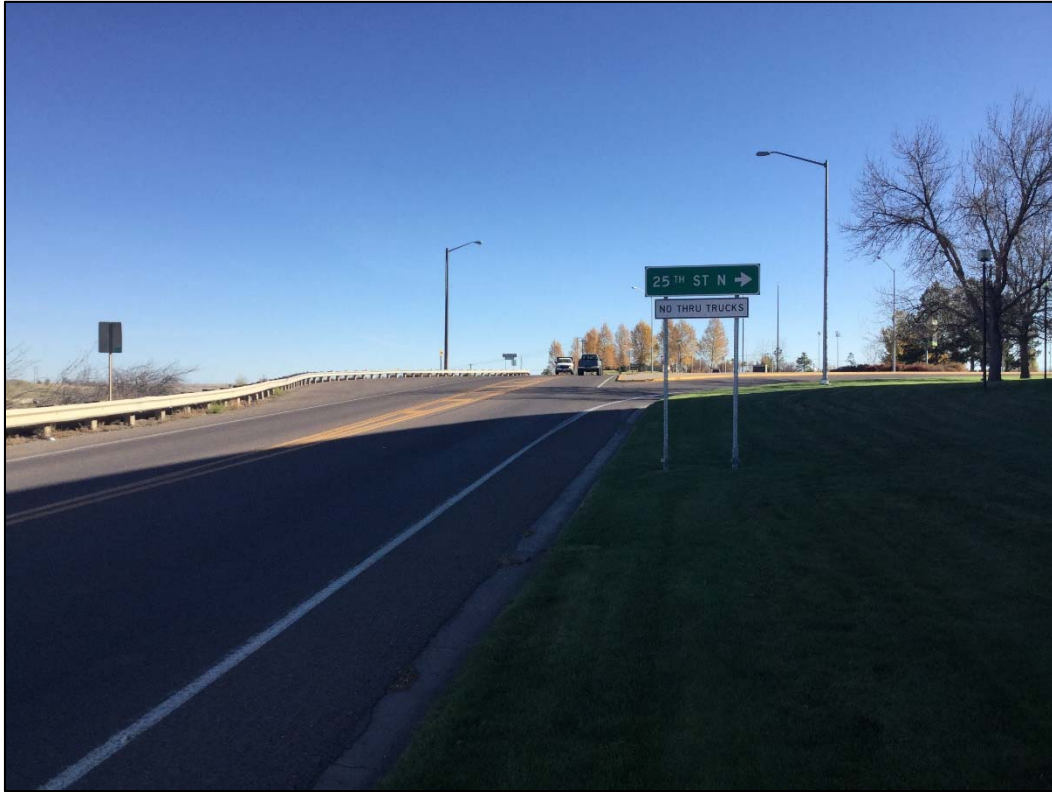
Photo 16: Looking east at the intersection with 25 th Street North (RP 4.2)
