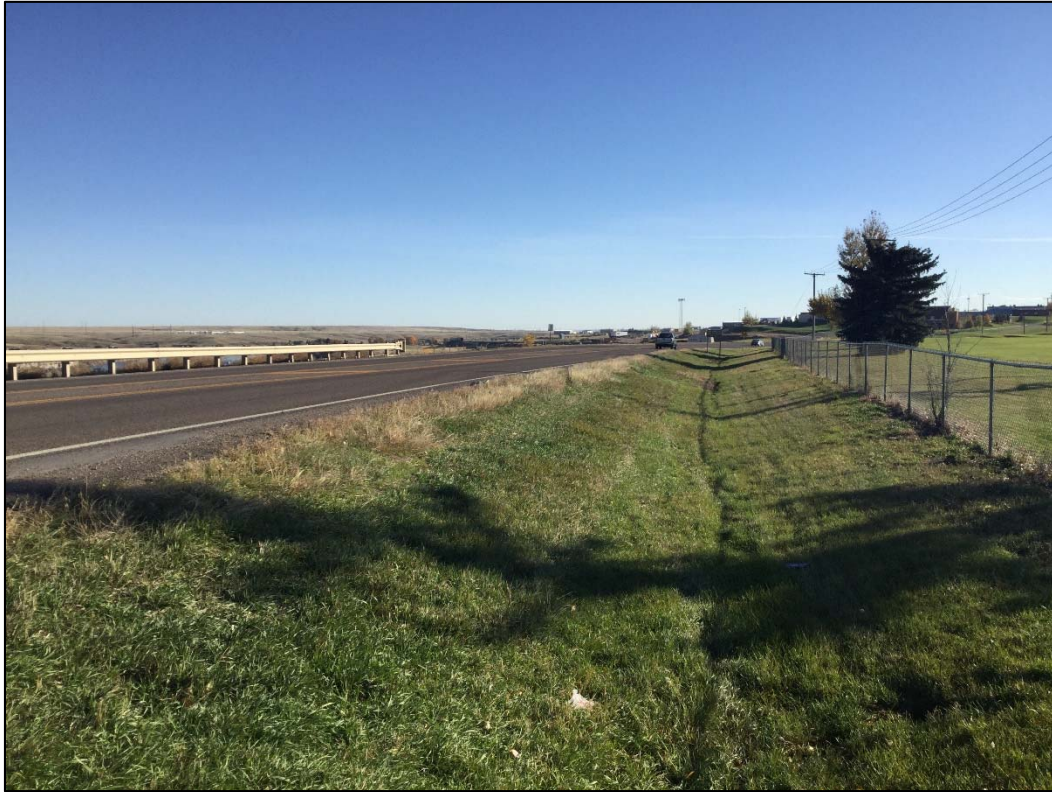
Photo 26: Looking east near Eagle Falls Golf Club (RP 4.8)
