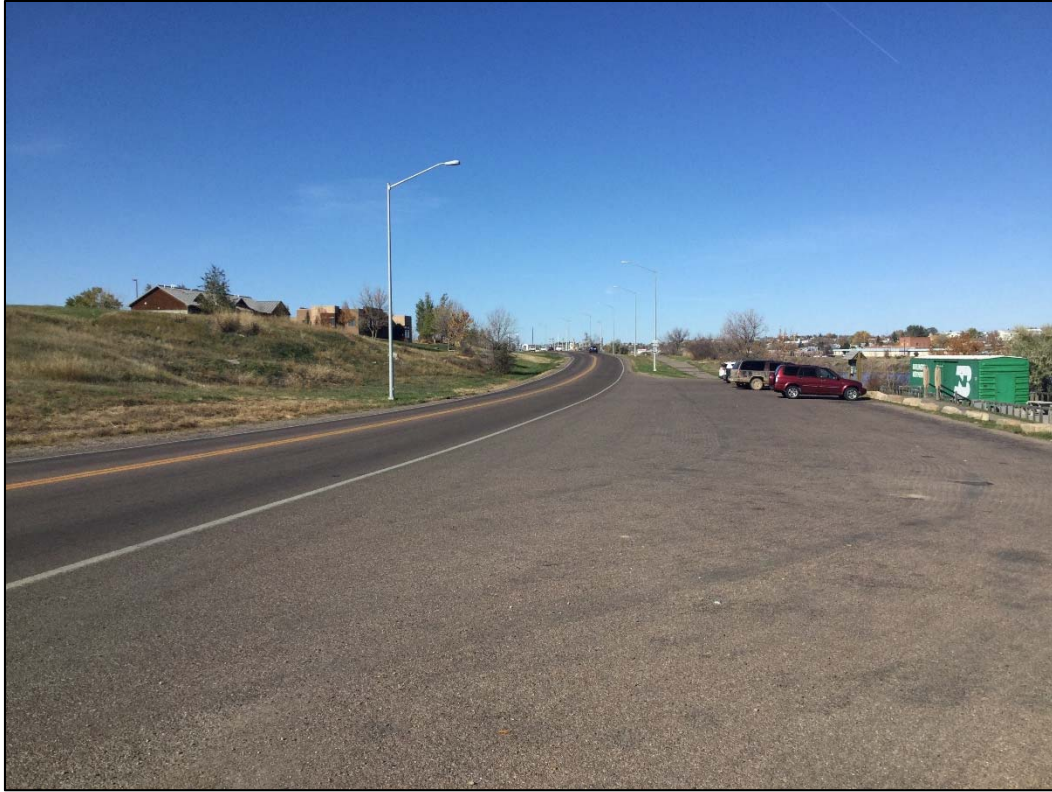
Photo 7: Looking west at the Caboose Trailhead (RP 3.8)
