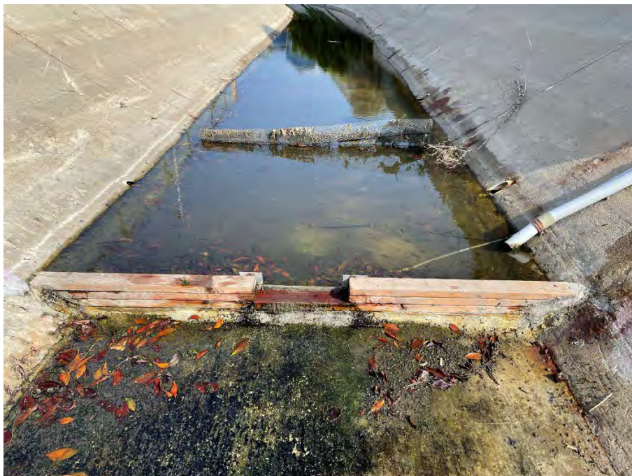
Figure 4-3. Rectangular Weir
