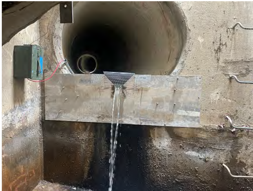
Figure 4-2. V-notch Weir on Outfall
