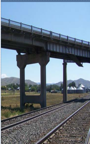
Looking east at MRL Railway and private land.
