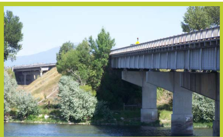
Looking northeast at MRL Bridge and Missouri River Bridge.
