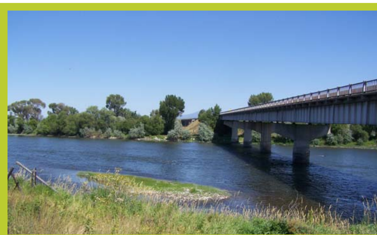
Looking northeast at Missouri River.
