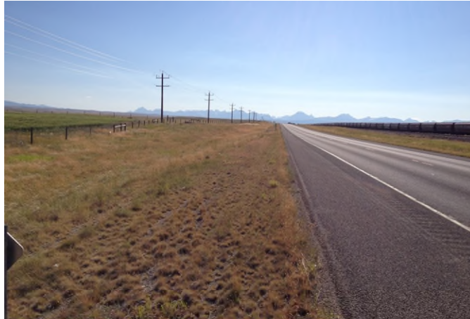
Photo 55. Segment 2, RP 231.1±, looking westbound.
