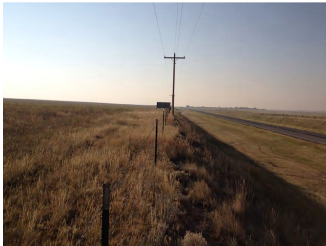
Photo 72. Segment 3, RP 282.1±, looking eastbound from north side of US 2.
