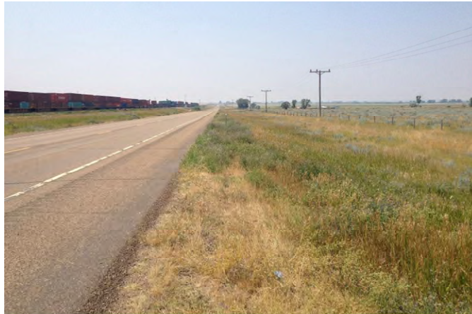
Photo 129. Segment 5, RP 511.8±, looking westbound.
