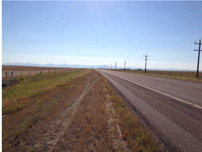
Photo 64. Segment 2, RP 241.4±, looking westbound.
