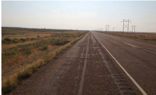
Photo 155. Segment 6, RP 574.7±, looking westbound.
