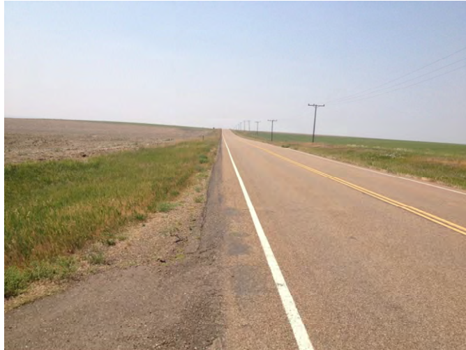
Photo 123. Segment 5, RP 505.5±, looking westbound.
