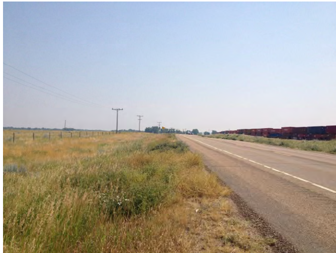
Photo 130. Segment 5, RP 511.8±, looking eastbound.
