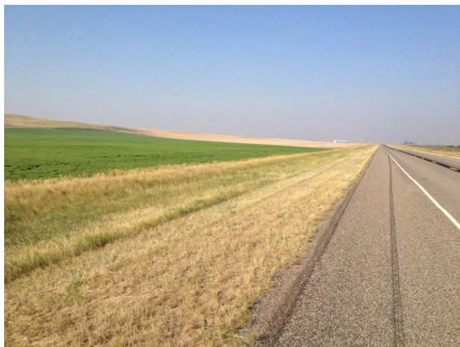
Photo 99. Segment 3, RP 312.0±, looking westbound.
