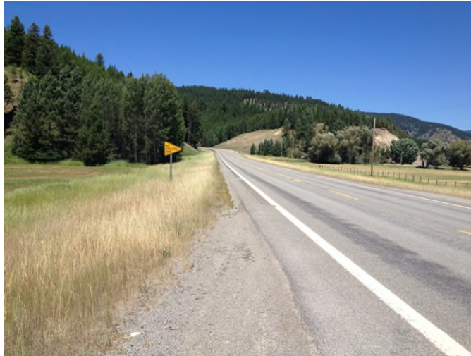
Photo 1. Segment 1, RP 55.8±, looking westbound.
