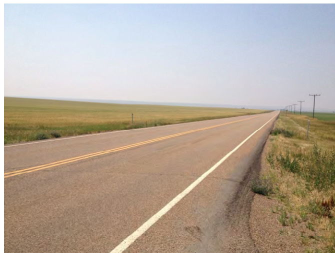
Photo 119. Segment 5, RP 503.5±, looking westbound.
