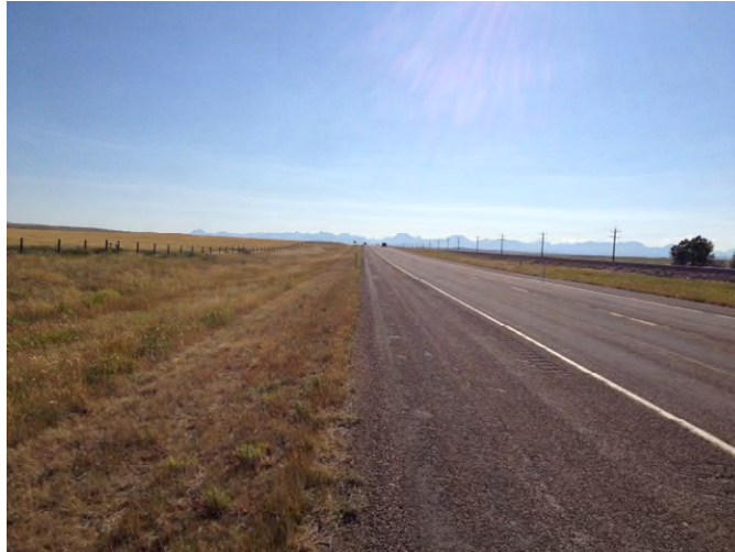
Photo 61. Segment 2, RP 237.2±, looking westbound.
