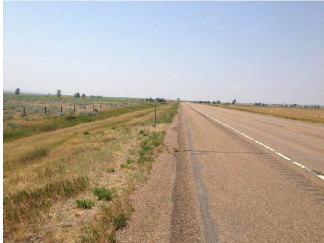
Photo 141. Segment 5, RP 522.8±, looking westbound.
