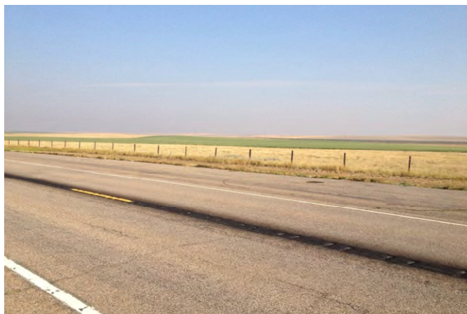
Photo 93. Segment 3, RP 300.8±, looking NW of US 2.
