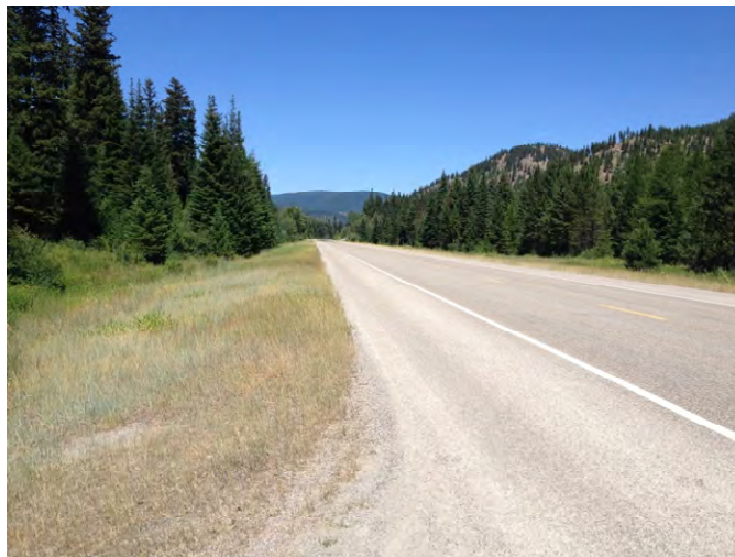
Photo 5. Segment 1, RP 58.3±, looking westbound.
