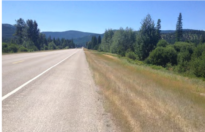
Photo 13. Segment 1, RP 62.2±, looking westbound.
