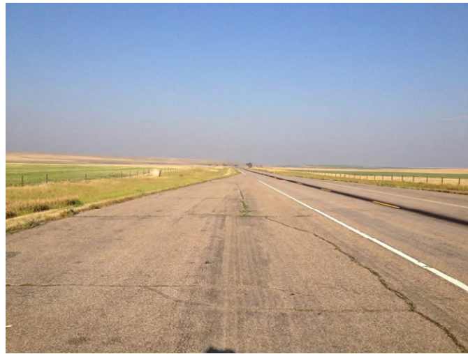
Photo 89. Segment 3, RP 300.8±, looking westbound.
