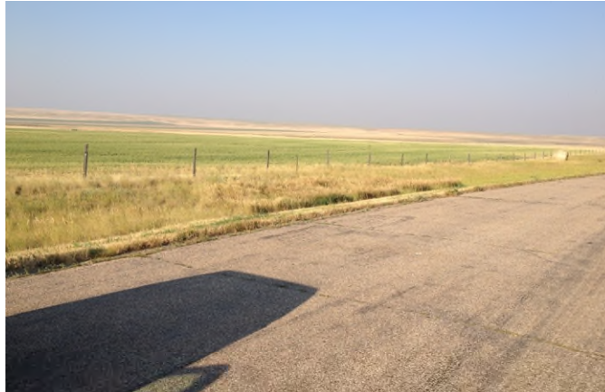
Photo 91. Segment 3, RP 300.8±, looking SW of US 2.
