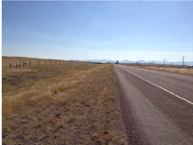
Photo 58. Segment 2, RP 235.9±, looking westbound.
