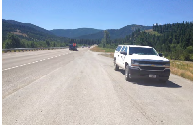
Photo 10. Segment 1, RP 61.5±, looking westbound.
