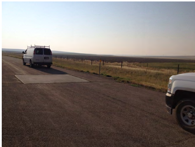
Photo 92. Segment 3, RP 300.8±, looking SE of US 2.
