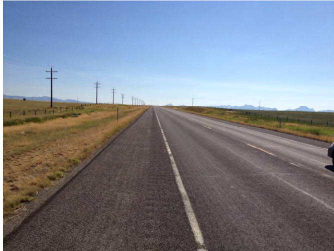
Photo 49. Segment 2, RP 227.9±, looking westbound.
