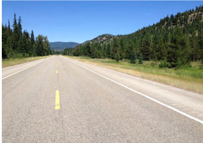
Photo 7, Segment 1, RP 58.5±, looking westbound.
