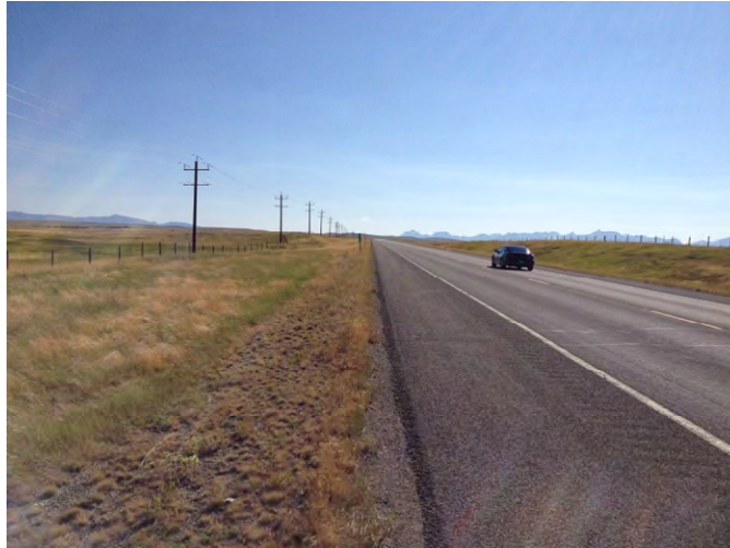
Photo 43. Segment 2, RP 226.0±, looking westbound.
