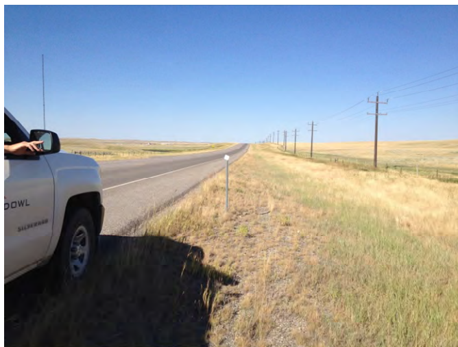
Photo 44. Segment 2, RP 226.0±, looking eastbound.
