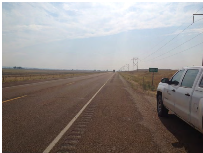
Photo 160. Segment 6, RP 581.1±, looking westbound.
