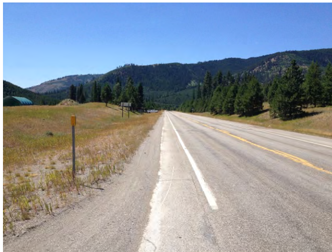
Photo 23. Segment 1, RP 66.5±, looking westbound, across from Forest Rd #6734.
