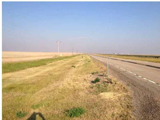
Photo 83. Segment 3, RP 293.9±, looking westbound.
