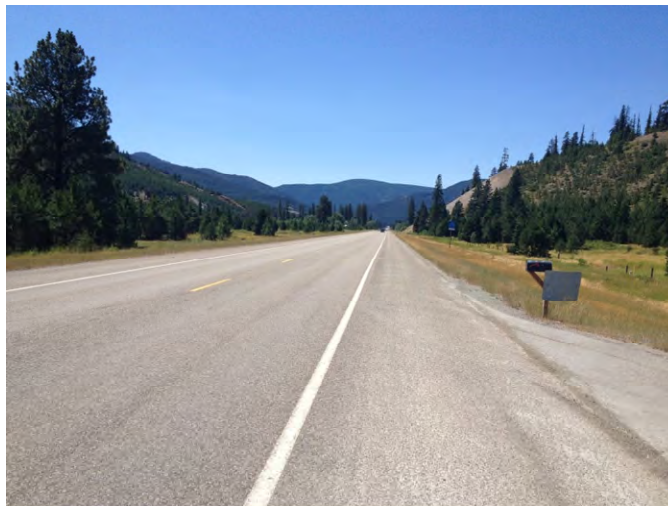
Photo 17. Segment 1, RP 63.1±, looking westbound.
