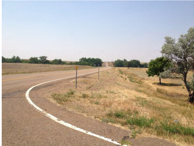
Photo 150. Segment 5, RP 527.3±, looking westbound from Vandalia Rest Area.
