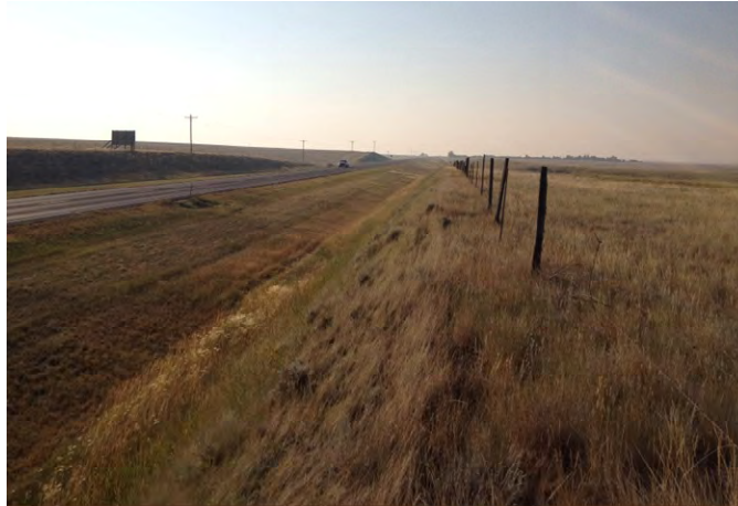
Photo 70. Segment 3, RP 282.1±, looking eastbound from south side of US 2.
