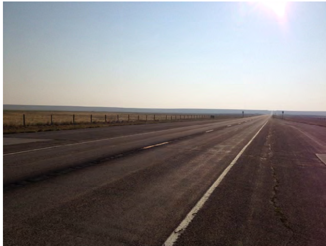
Photo 94. Segment 3, RP 300.8±, looking NE of US 2.
