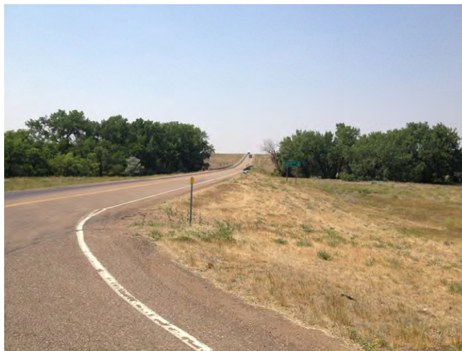
Photo 148. Segment 5, RP 527.1±, looking westbound from Vandalia Rest Area.
