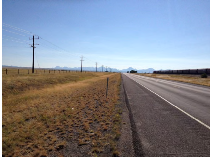
Photo 52. Segment 2, RP 230.4±, looking westbound.
