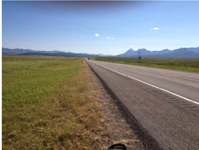
Photo 34. Segment 2, RP 213.9±, looking westbound.
