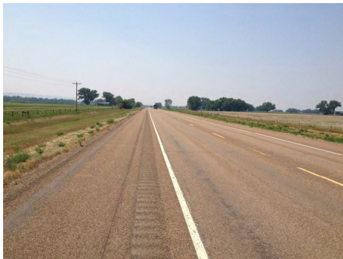
Photo 133. Segment 5, RP 516.1±, looking westbound.
