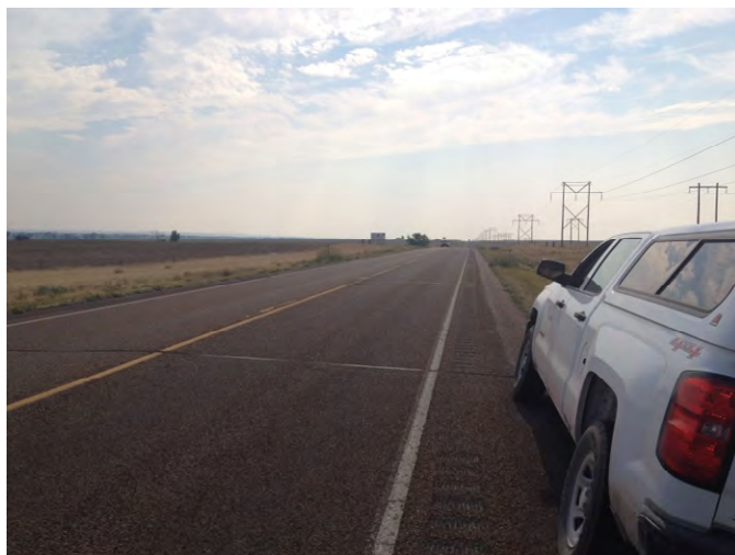
Photo 163. Segment 6, RP 585.4±, looking westbound.
