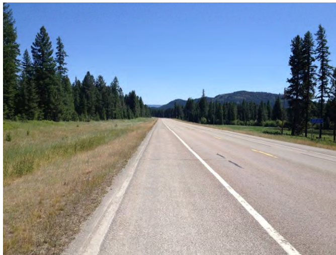
Photo 29. Segment 1, RP 75.2±, looking eastbound.
