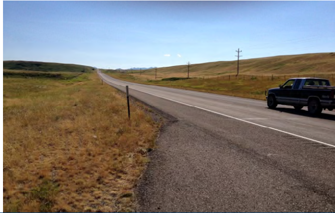
Photo 37. Segment 2, RP 218.7±, looking westbound.
