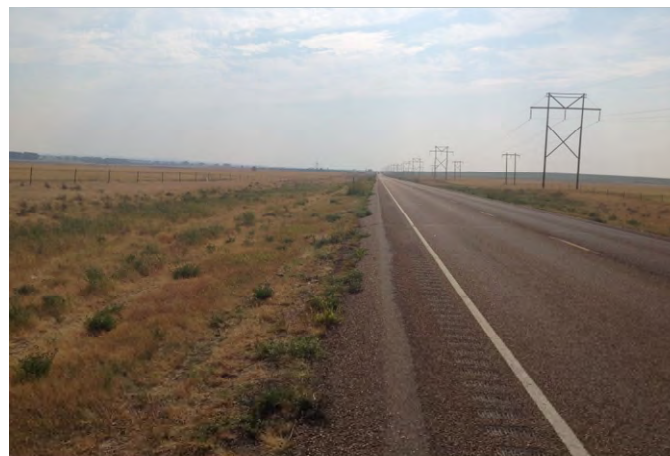
Photo 165. Segment 6, RP 586.9±, looking westbound.
