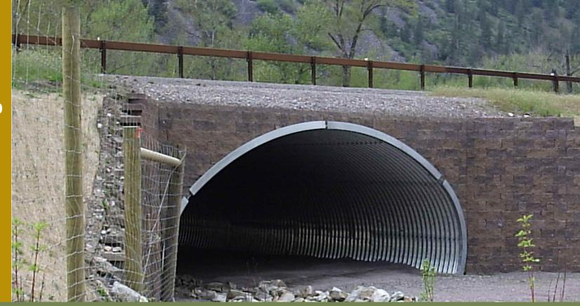
Wildlife fences are effective at reducing wildlife-vehicle collisions and improving road safety by keeping animals off highways. However, fencing alone can exacerbate habitat fragmentation and restrict wildlife movement. To mitigate this, fences should be paired with wildlife crossing structures—such as underpasses, overpasses, and jumpouts—to allow safe animal passage.
