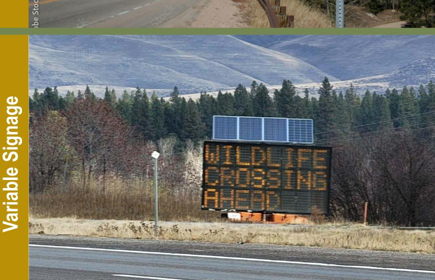
Variable, or dynamic, wildlife warning signs are more effective than static signs because they can be activated during specific time periods based on known wildlife movement patterns. By providing drivers with timely, location-specific alerts, these signs can significantly reduce wildlife-vehicle collisions, particularly in known crossing areas.
