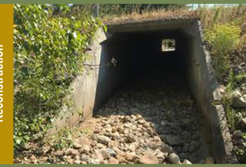
Rehabilitation or reconstruction of existing culverts can improve their suitability for wildlife passage by modifying their size, shape, or condition. Features such as ramps, wider openings, or natural substrates can be incorporated to enhance their effectiveness in attracting wildlife and facilitating safe crossings.
