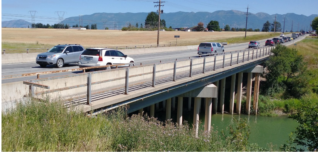
Stillwater River Bridge
