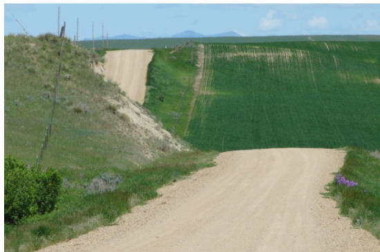
Figure 25: Combined horizontal/vertical curve and roadside obstruction south of Stulc Ln. (RP 31.5)
