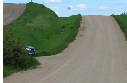
Figure 21: Restricted intersection sight distance at Stulc Ln. (RP 32.4)
