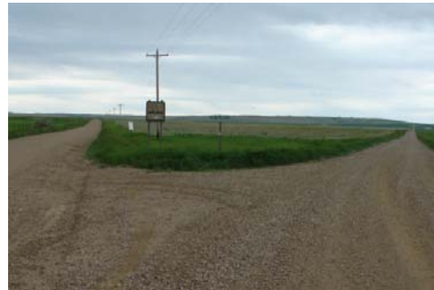
Figure 22: Skewed intersection at Eight Mile Bench Road (RP 59.4)
