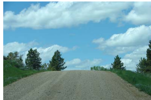
Figure 18: Vertical curve near RP 35.7
