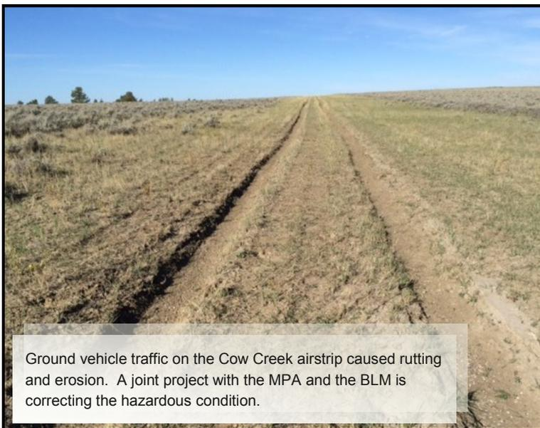
Ground vehicle traffic on the Cow Creek airstrip caused rutting and erosion. A joint project with the MPA and the BLM is correcting the hazardous condition.
