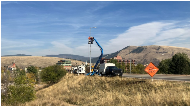
Pictured top right, bottom left: MDT installing traffic monitoring devices in Missoula.
