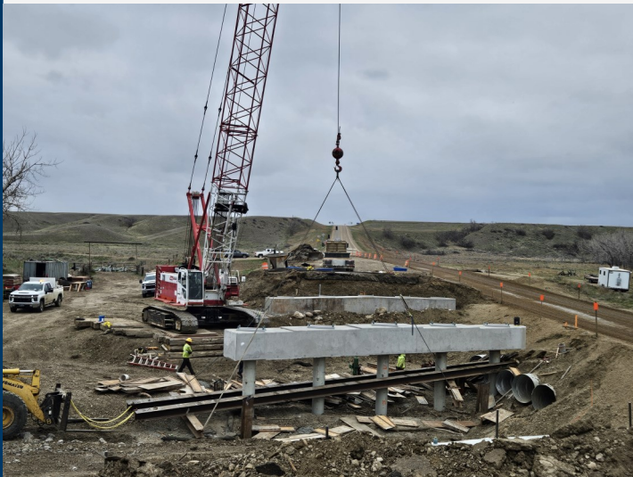
The completed piling and bridge caps on US 2 at Buggy Creek.
