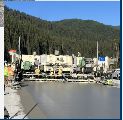
Pictured to the right is a smooth mat of new concrete, the finished product produced by the automated paver and placer.
