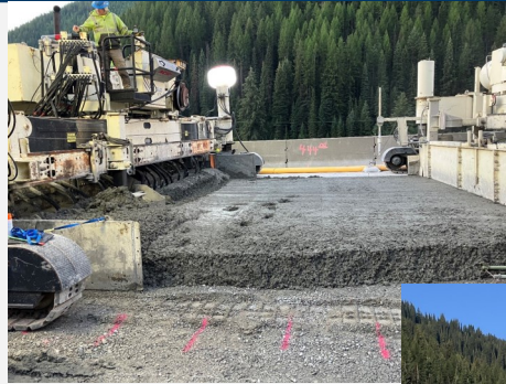
Pictured to the left is the automated paver used for this project, smoothing the concrete out to place it at the correct thickness.
