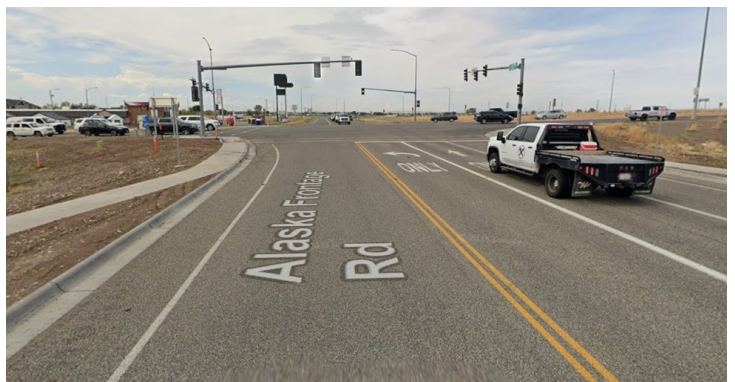
Pictured above is the dedicated west-bound left turn lane added at the Alaska Frontage Road and Jackrabbit Lane intersection as part of the West Post Development project.
