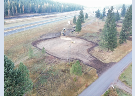
Picture by Jon Schwarder, Reed Mountain Construction
