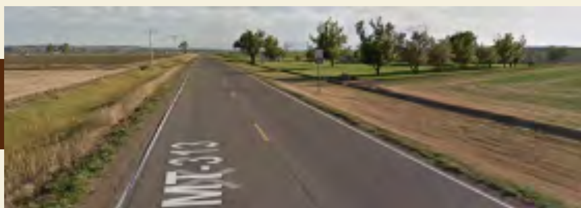
Example road before widening
