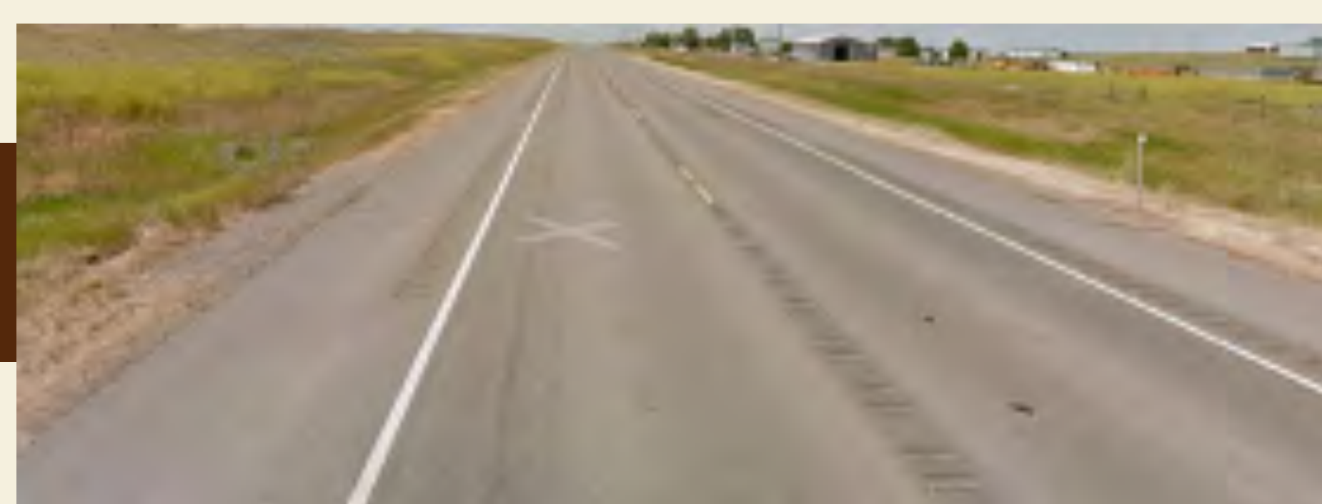
Example road after widening
