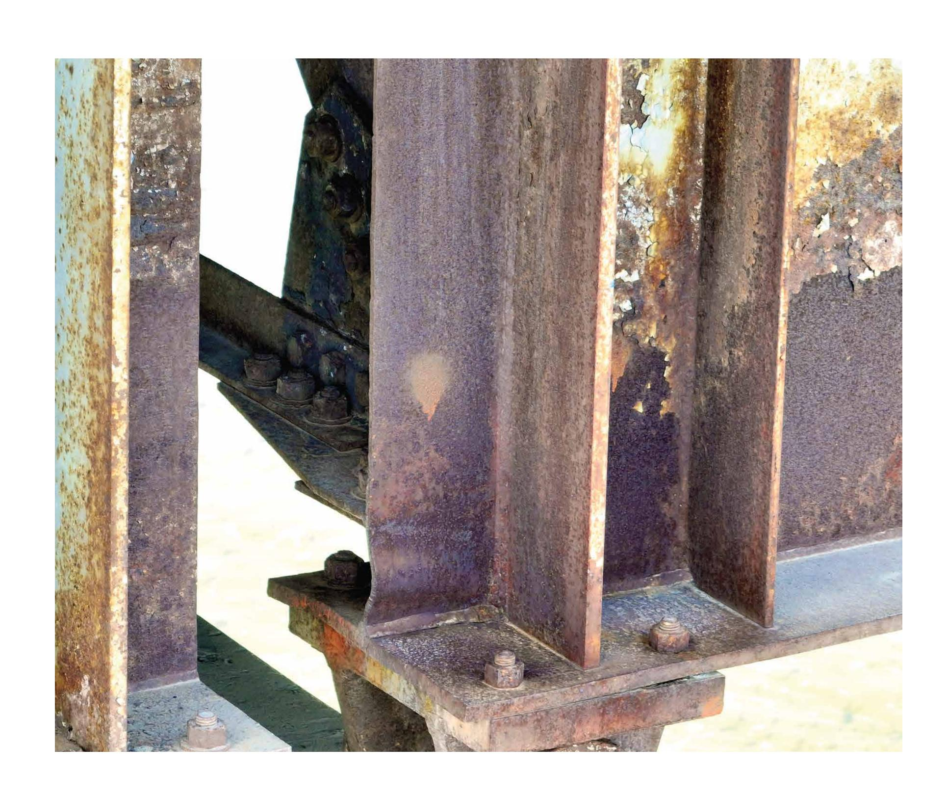
In order to repair the girders, jacks will be placed in-between girders, next to the bearings, to raise the structure.
