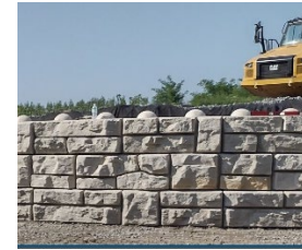
CONSTRUCT RETAINING WALLS
