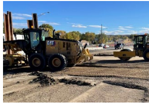
ROAD AND DITCH GRADING
